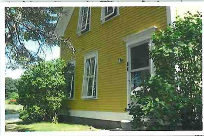
Recommended Historic exterior storm windows have been well maintained and continue to perform as intended.
