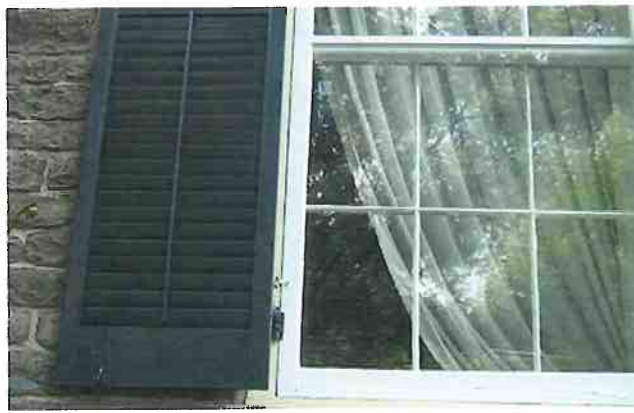
Recommended Historic exterior storm windows have been well maintained and continue to perform as intended.
