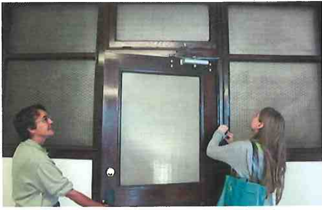
Recommended The wall and door glazing ensures that the corridor receives natural daylight and the operable transom helps air to circulate in this historic office building.
