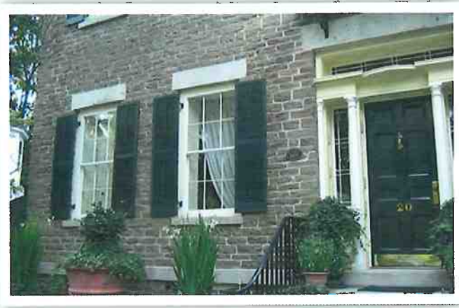
Recommended Historic exterior storm windows have been well maintained and continue to perform as intended.
