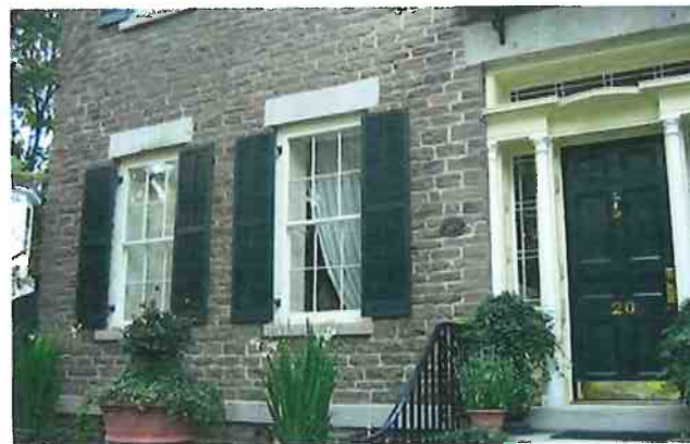
Recommended Historic exterior storm windows have been well maintained and continue to perform as intended.
