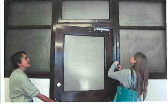
Recommended The wall and door glazing ensures that the corridor receives natural daylight and the operable transom helps air to circulate in this historic office building.
