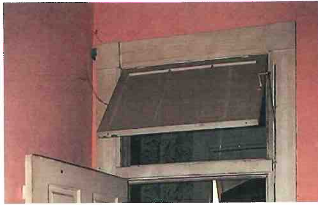
Recommended Transoms and screen doors are distinctive and practical features that provided cross ventilation in this historic hotel.
