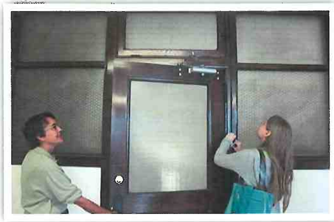
Recommended The wall and door glazing ensures that the corridor receives natural daylight and the operable transom helps air to circulate in this historic office building.
