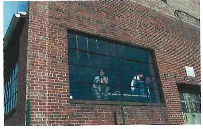
Recommended Original metal windows were appropriately repaired as part of the rehabilitation of this historic industrial building. After rehabilitation.
