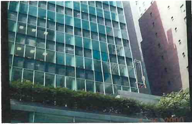
Recommended The original windows, which were deteriorated beyond repair, featured a dark tint. They were replaced with a slightly lighter-tinted glazing to improve daylighting in this mid-century modern office building.
