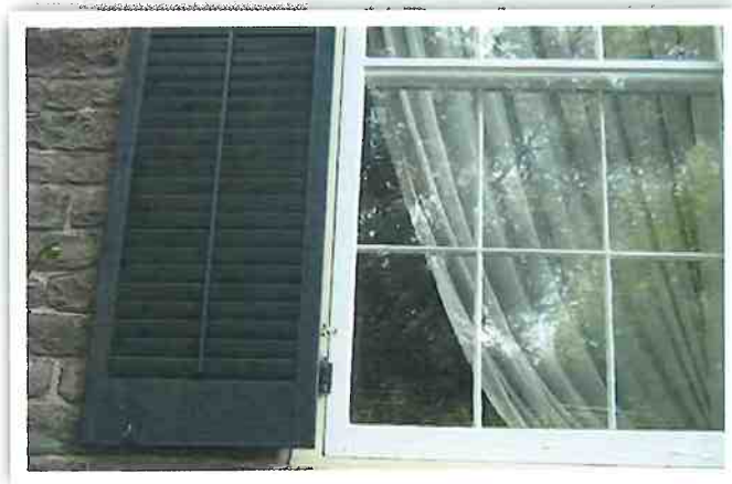
Recommended Historic exterior storm windows have been well maintained and continue to perform as intended.
