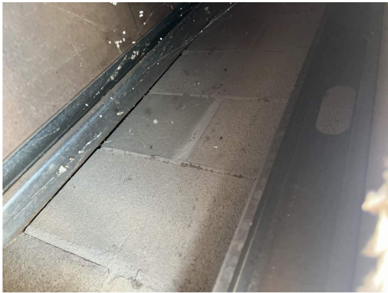
③ DROP 2 - VERTICAL STUDS INSIDE PILASTER ATTACHED TO THE SUPPORTING CMU WALL
