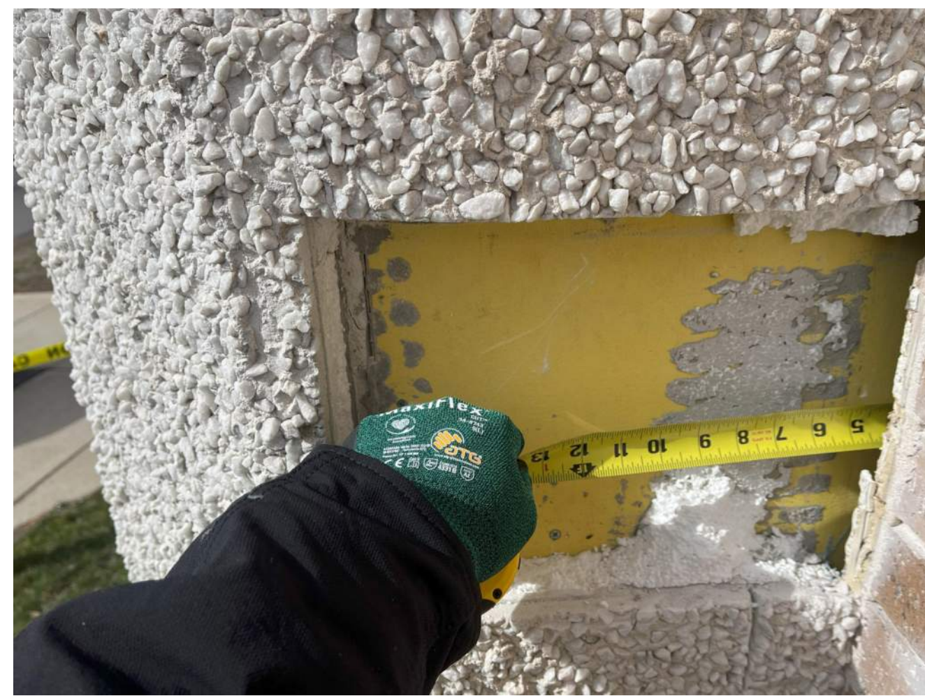
16 DROP 1 - FACE OF THE BRICK TO THE WALL GYP BOARD
