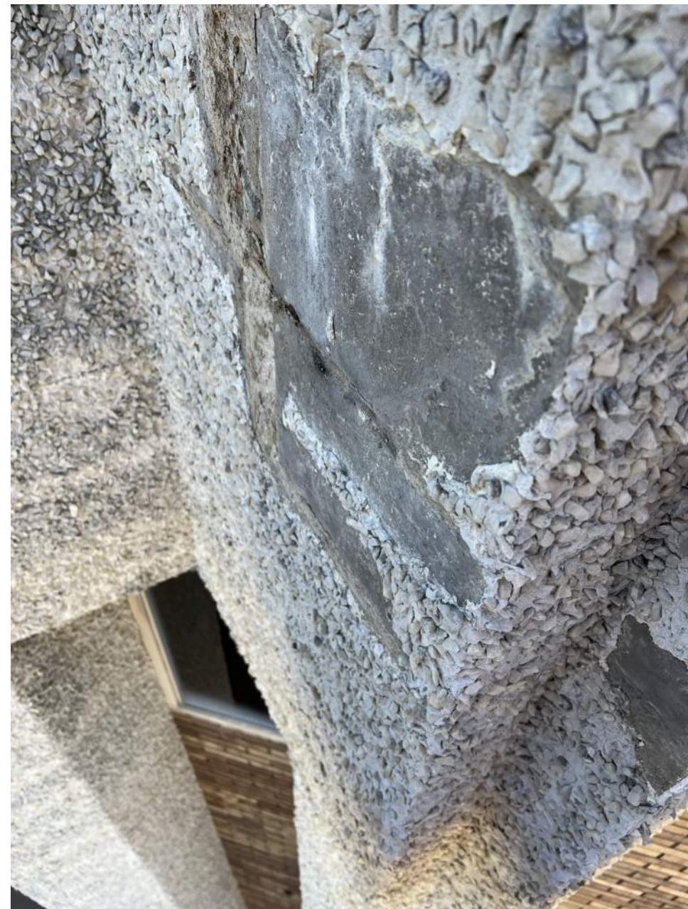
7 STUCCO CRACKING AND SPALLING AT ROOF LEVEL
