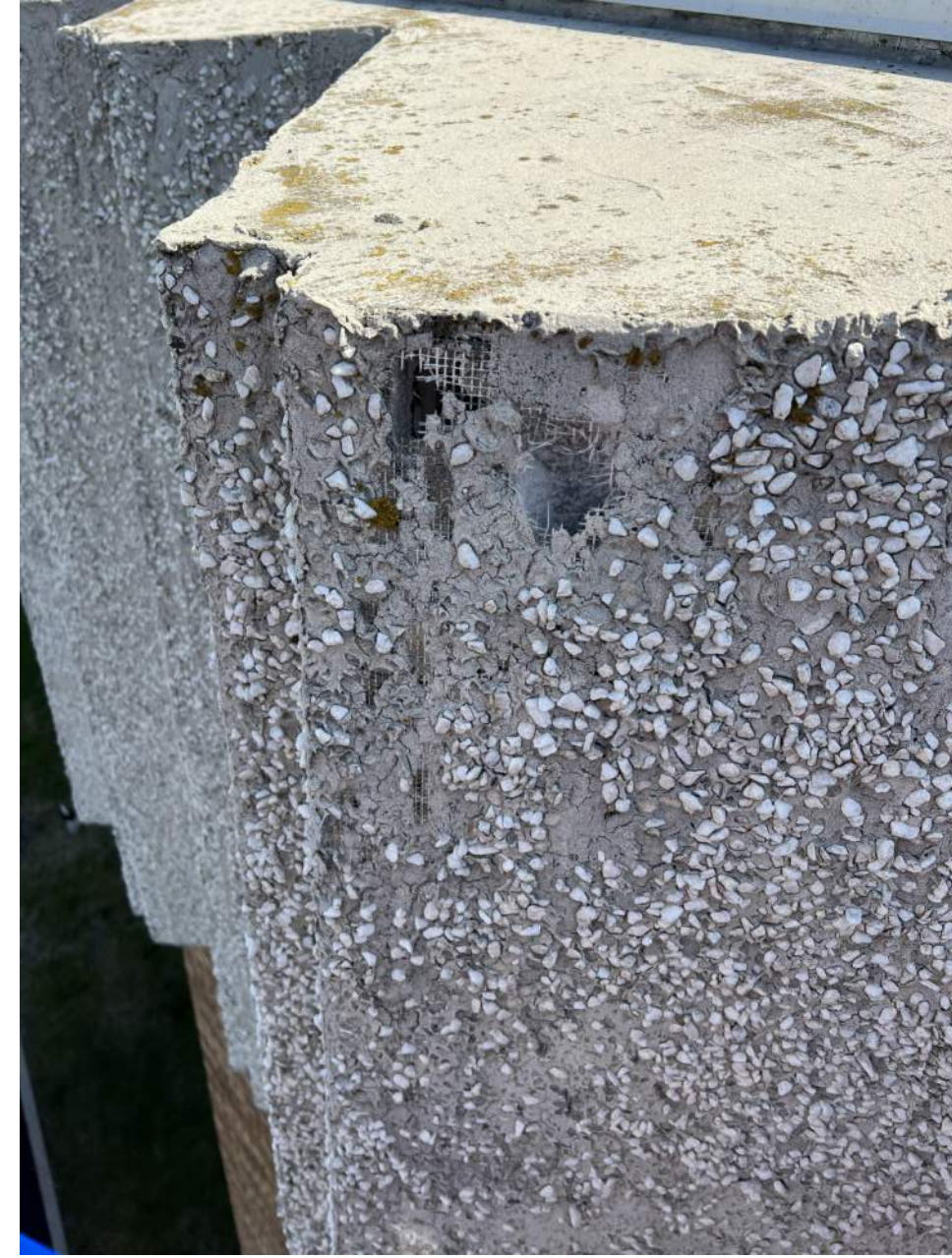
8 SHOWING DAMAGE TO RIGID INSULATION SUBSTRATE
