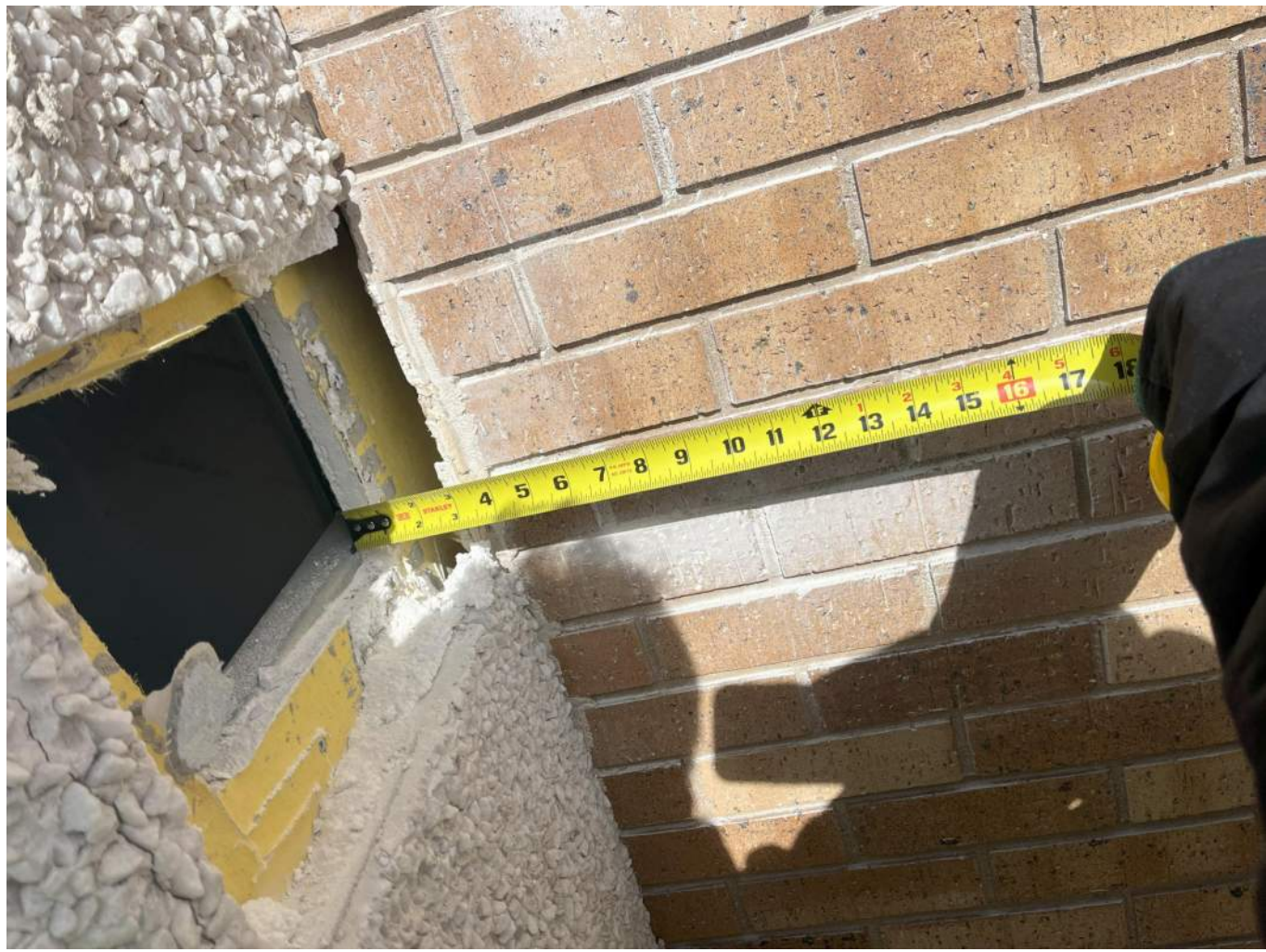
① DROP 1 - PILASTER SKIN THICKNESS
