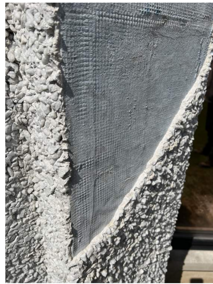
11 STUCCO DETACHED FROM SUBSTRATE SGOWING CMU SUBSTRATE
