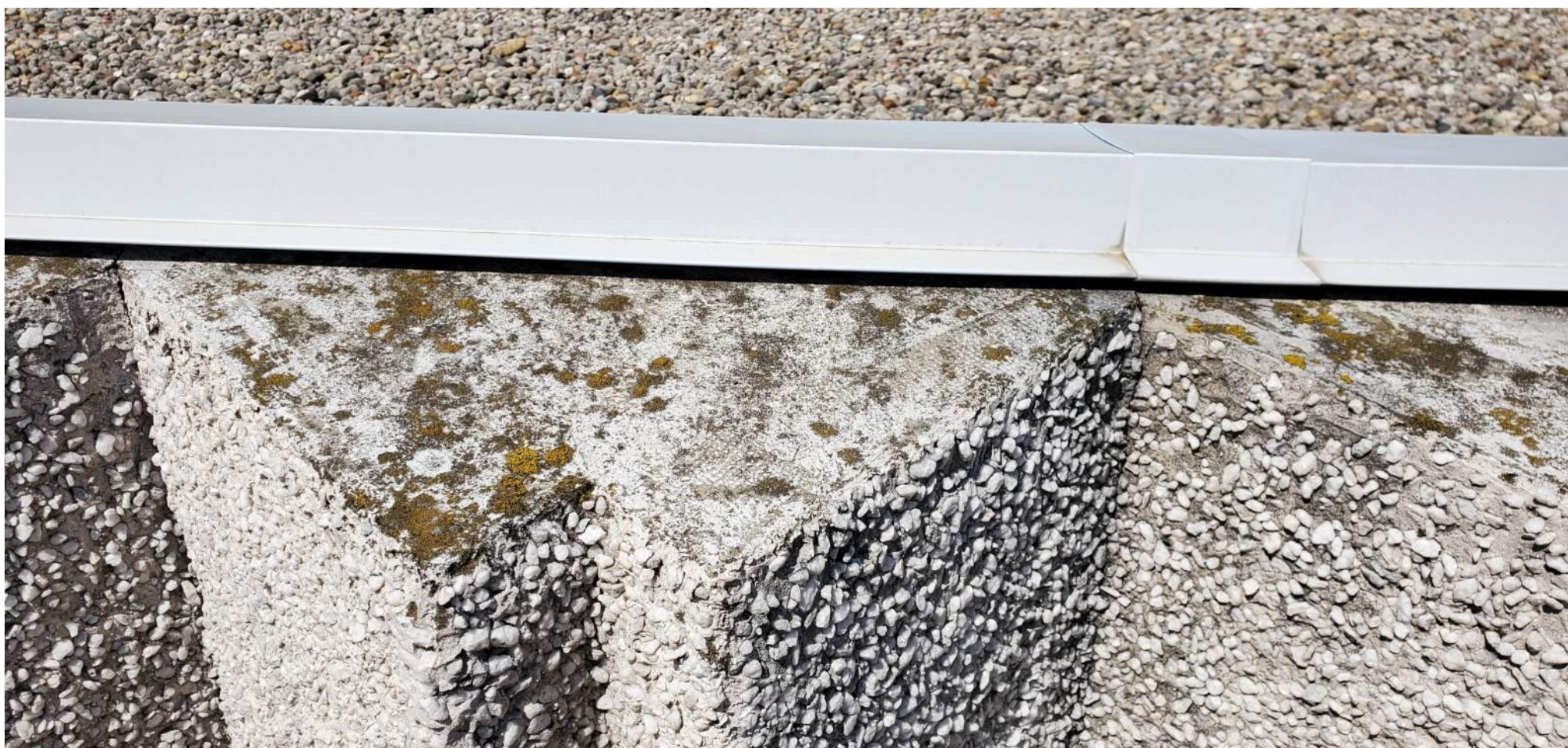
9 STUCCO DELAMINATING AT ROOF LEVEL
