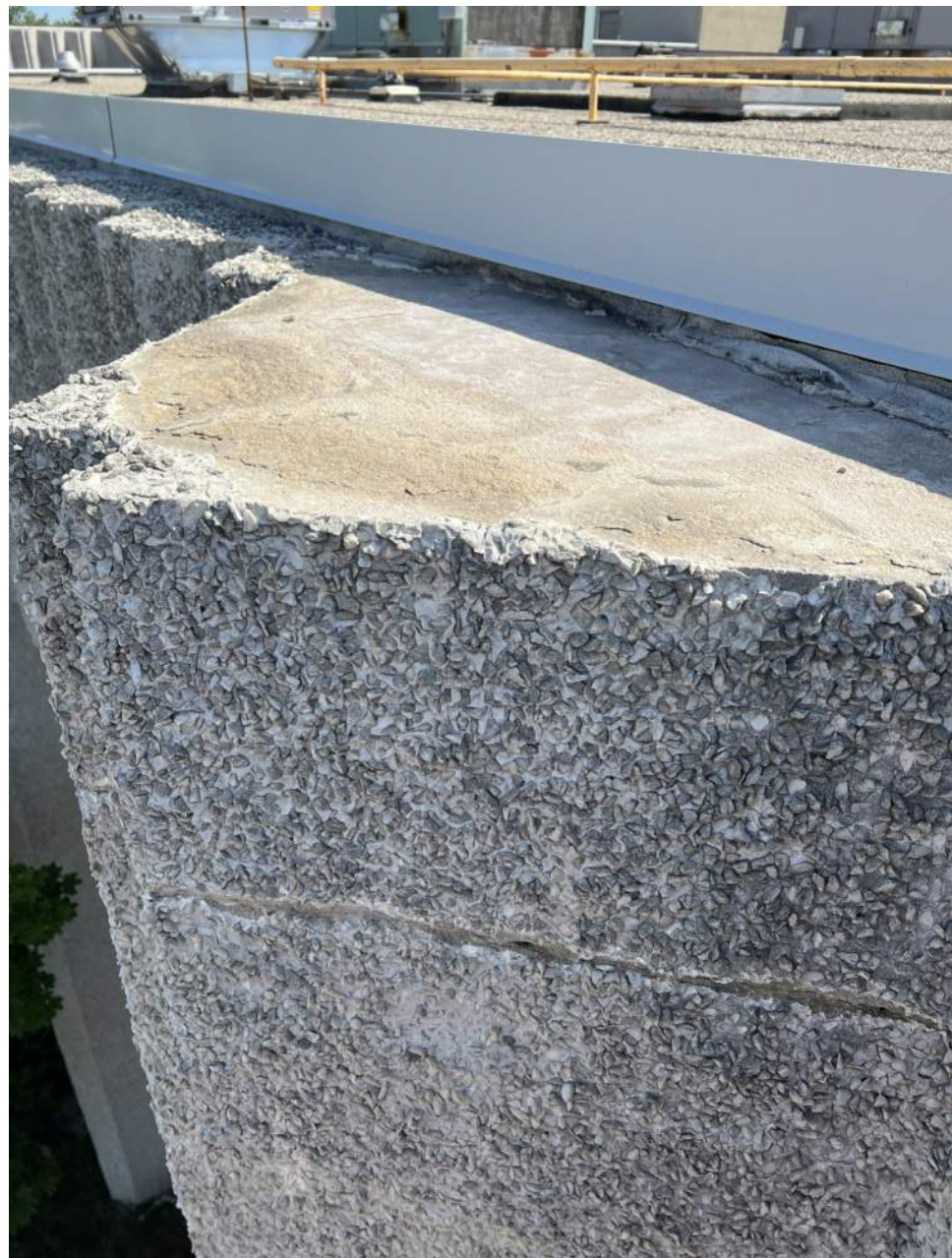
6 STUCCO ALMOST COMPLETELY MISSING AT ROOF LEVEL
