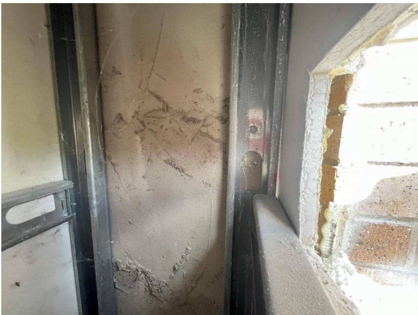
14 DROP 1 - PILASTER LAYERS AND VERTICAL STUDS INSIDE
