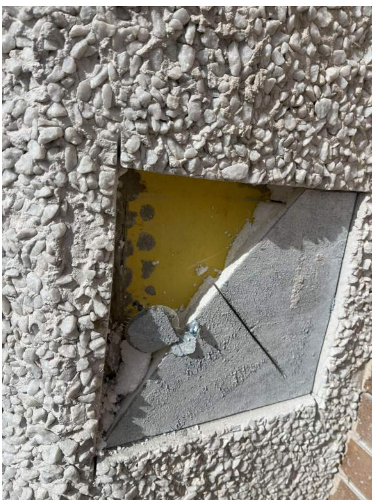
13 DROP 1 - EXTERIOR LAYERS DOWN TO GYP BOARD
