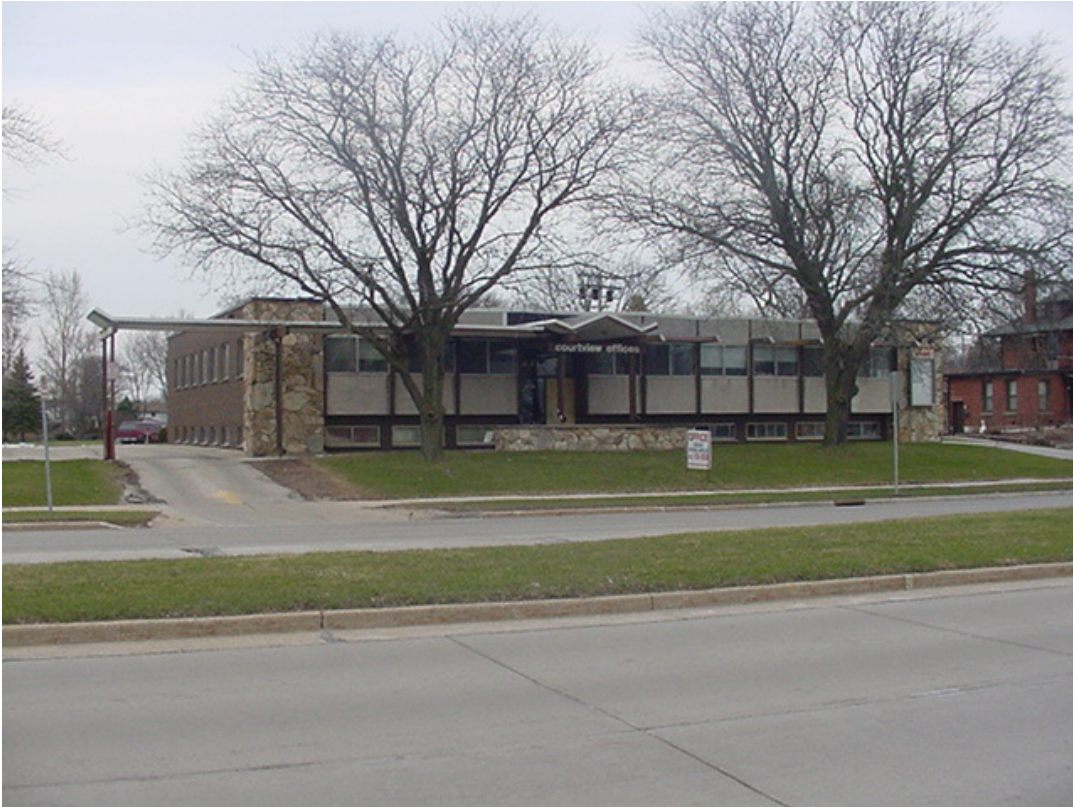
No. 1: Existing South (Front) Elevation: Replace windows with dark bronze frames and tinted glass; Remove vertical wood columns between windows; Remove Wood Sun Shade above windows; Replace Stucco with EIFS (See New South Elevations).
