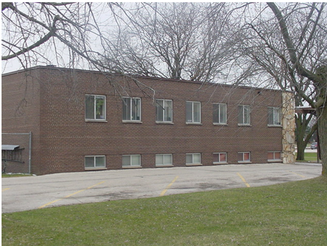
No. 10 Existing West Elevation: Remove existing windows and replace with bronze frames and tinted glass and no other changes.
