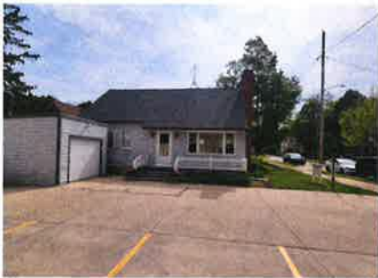
West Elevations: Carroll University Public Safety House. House siding is wood, garage siding is vinyl.
