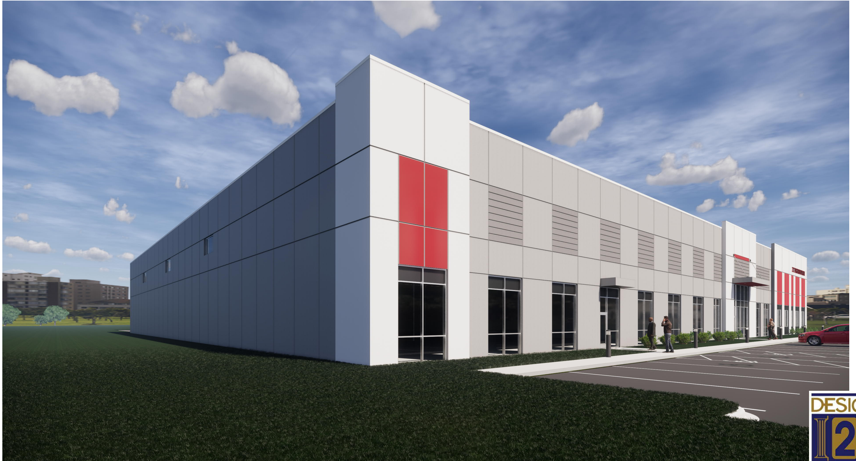
VIEW FROM NORTHEAST CORNER
