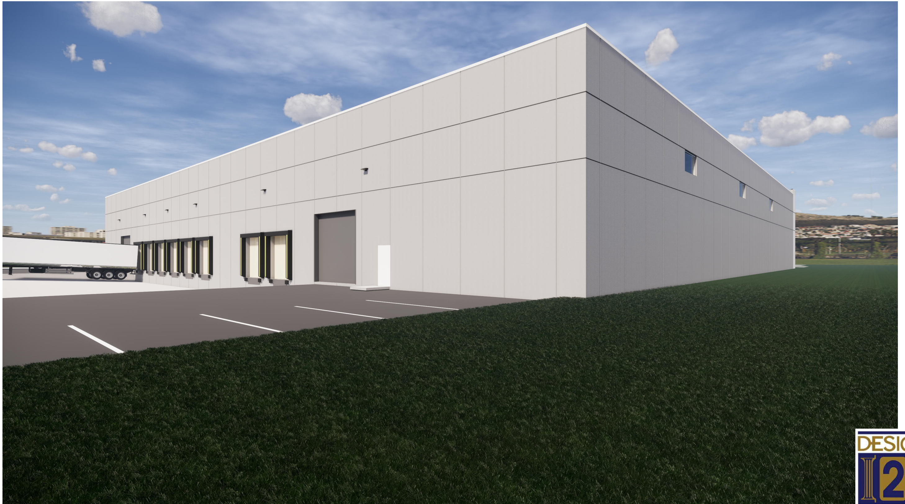
VIEW FROM SOUTHEAST CORNER
