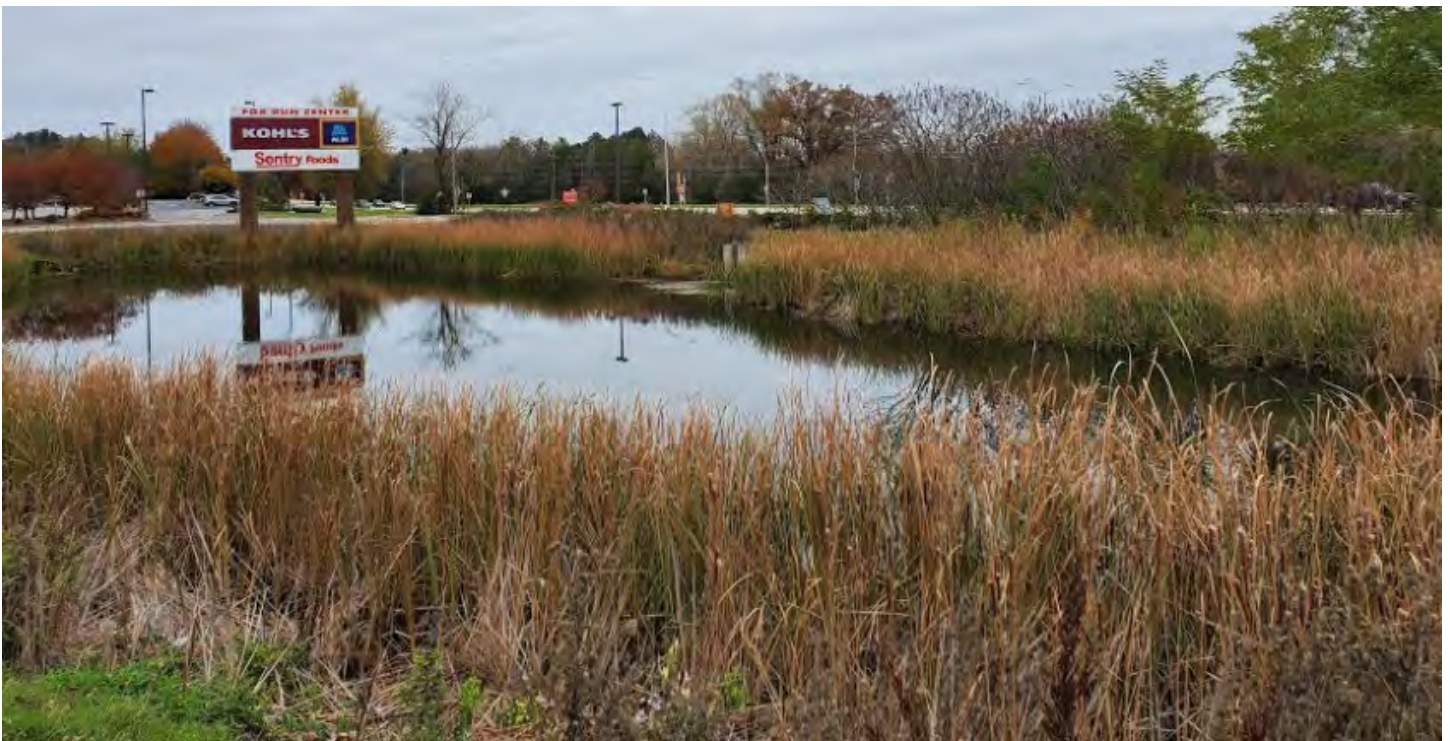
10- Standing south of the stormwater pond facing northeast.
