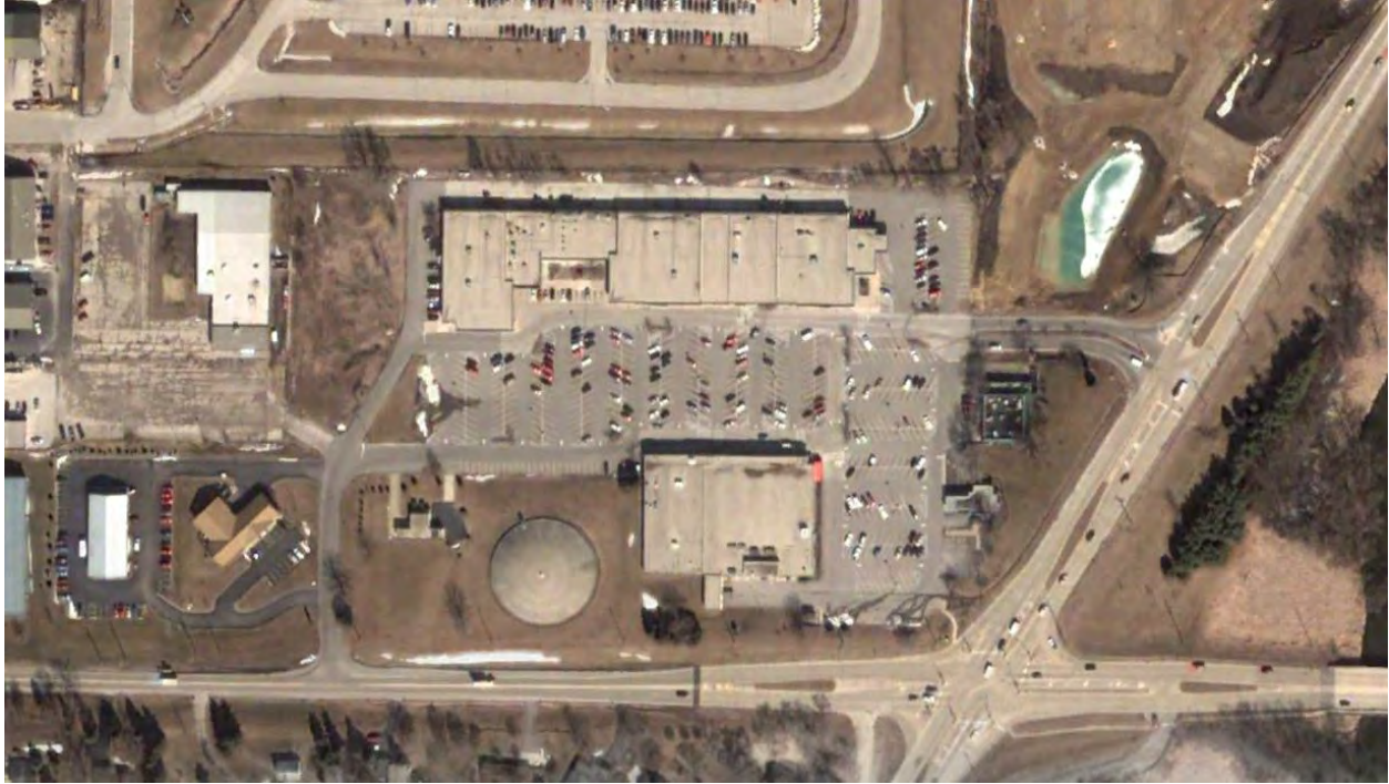
2002- A pond was constructed in the northeast corner of the Site.
