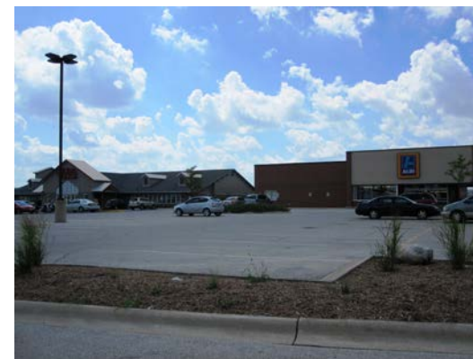
Aldi & Golden Corral on remediated landfill site
