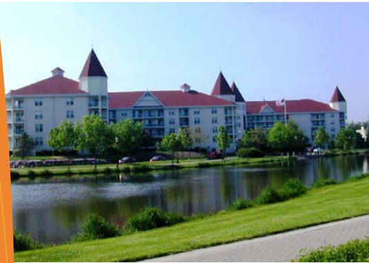
River's Edge Apartments
