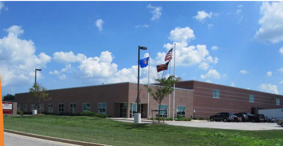
Gaco Western Relocation & Expansion
