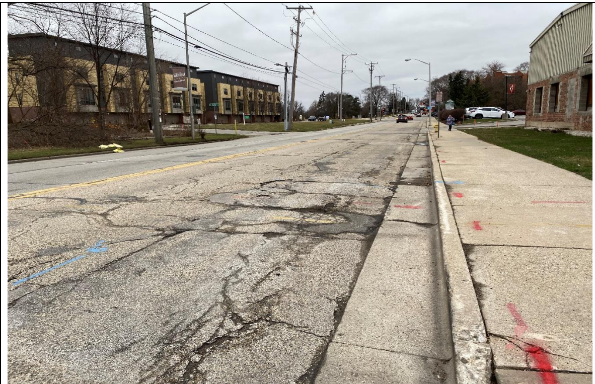
LOOKING WEST ON WEST ST. PAUL AVENUE
