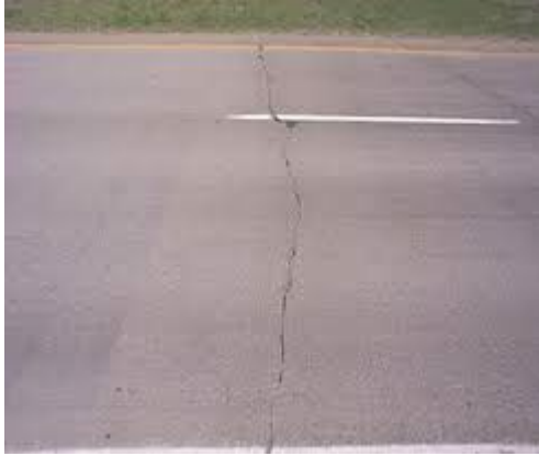
Slab Cracking
