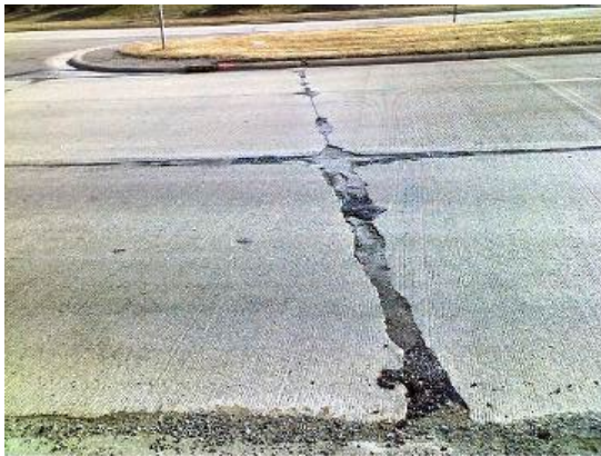
Joint Spalling/Failure
