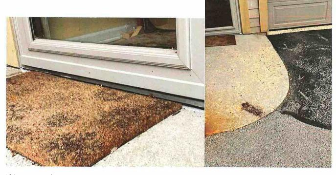
This concrete damage extends into my entry, affecting the door frame and openings, creating damage to the garage entry, and degrading the concrete surface down to the foundation level, allowing water to seep into the garage. The board voted to have the concrete repaired back in 2018/2019, but the vendor never completed the work, I think he developed medical issues. There are drafts and moisture, it expands and contract thru the seasons. It is unsightly.
