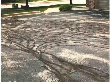
In addition to the destruction of the concrete surface at the entry to my garage and around the entry ways, the asphalt is in complete disarray. The entry to the garage was patched in order to address the irregularity causing standing water that freezes at the entry surfaces in front of the garage during the winters, and the salt used destroyed the concrete. Mine sustained the most damage on the property. The gutters overflow and create a waterfall, contributing to the staining and degradation.
