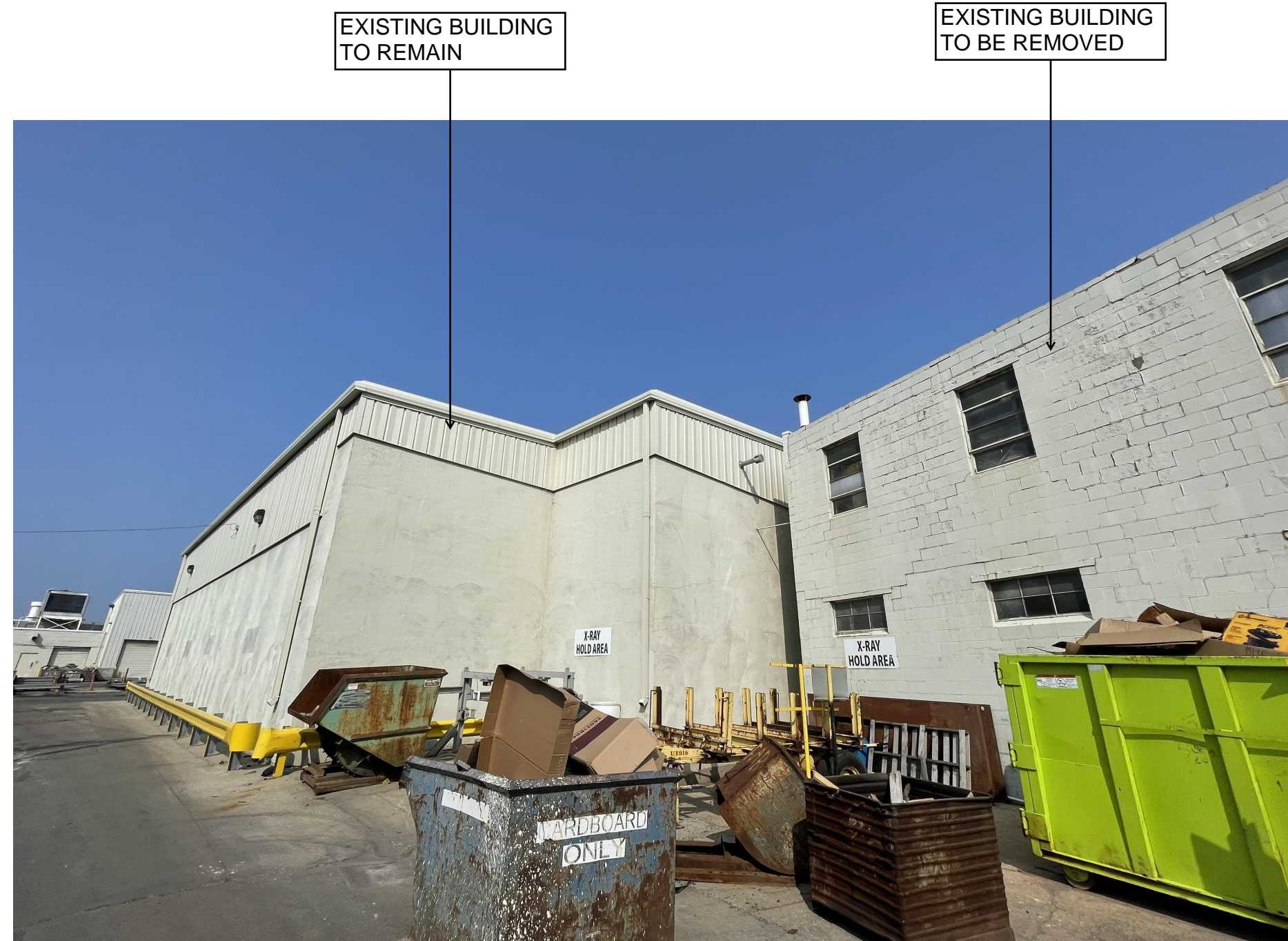
EXISTING BUILDINGS - VIEWED FROM SOUTHEAST
