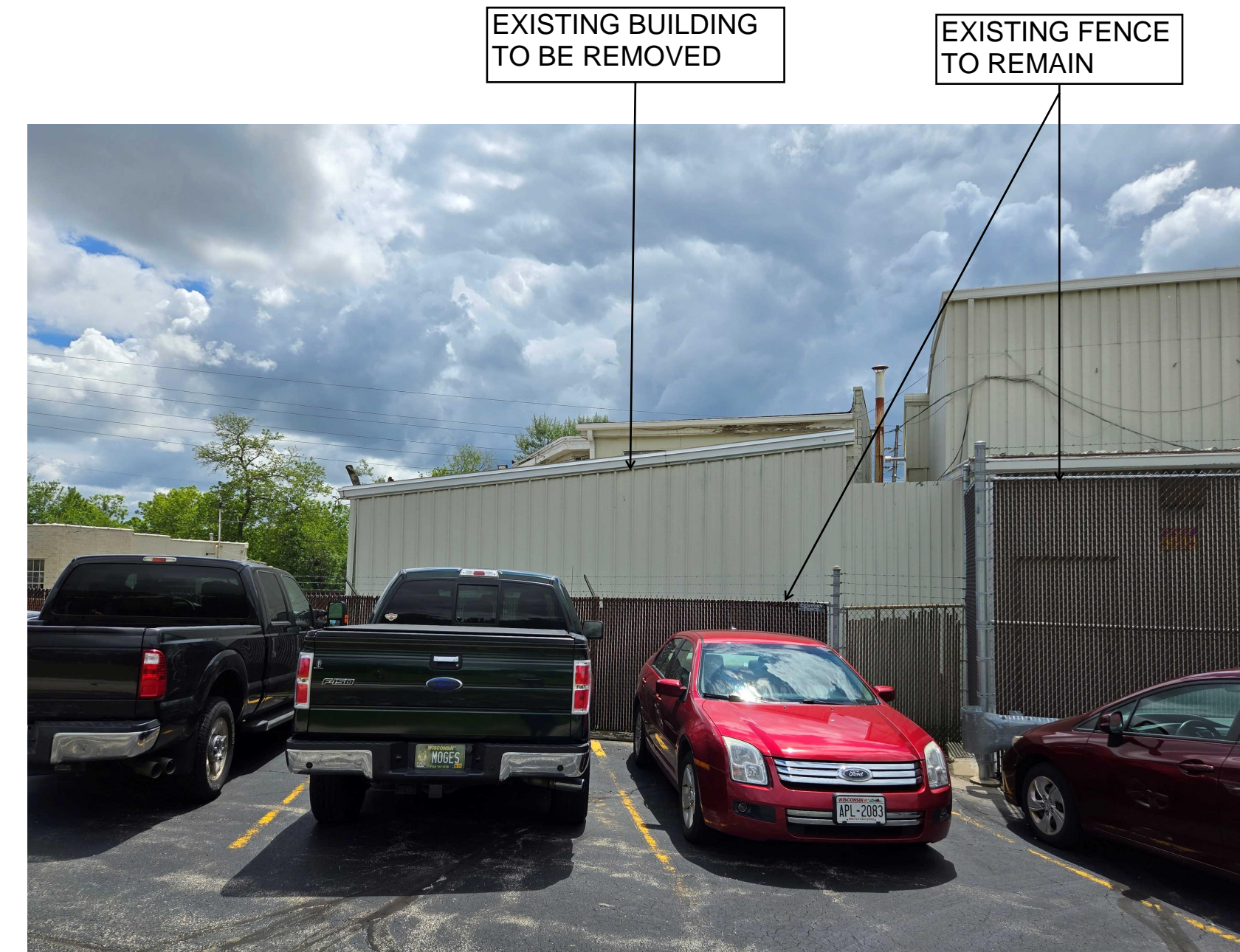
EXISTING BUILDING & FENCE - FACADE FACING ST PAUL
