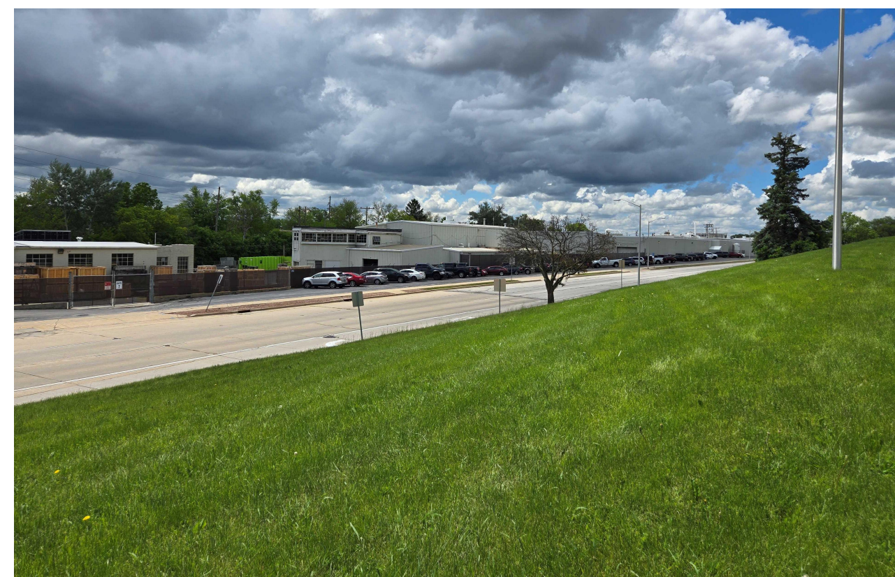
EXISTING BUILDINGS - VIEWED FROM ST PAUL HEADING SOUTHWEST
