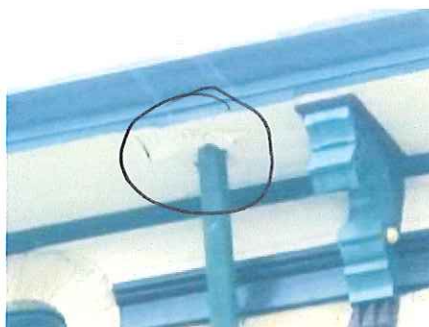
Figure 7: The soffit board above the downspout on the upper north side of the home shows evidence of wood rot.
