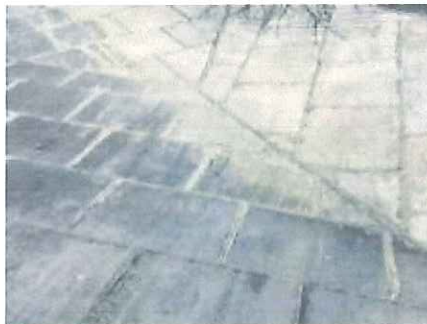
Figure 12: The front porch roof has seams that need to be caulked or sealed.
