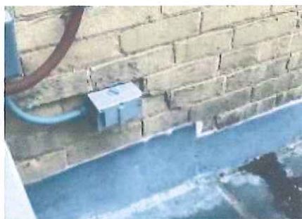
Figure 9: Slight shearing and loose mortar in the joints is visible in the brick behind the AC units on the balcony.
