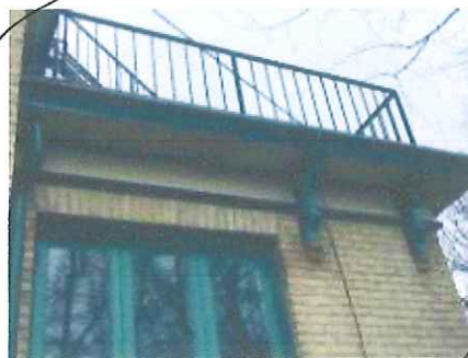
Figure 8: The soffit on the south side of the home near the southeast corner shows evidence of wood rot.
