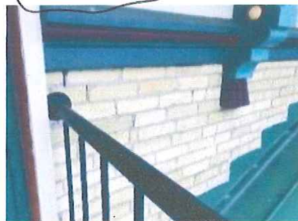
Figure 10: Loose mortar joints visible in the brick to the right of the entry door to the 3 rd floor kitchen.
