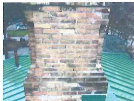
Figure 11: The right side chimney chase has several spots of loose or missing mortar in the brick joints.
