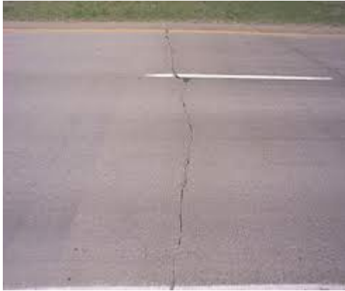
Slab Cracking
