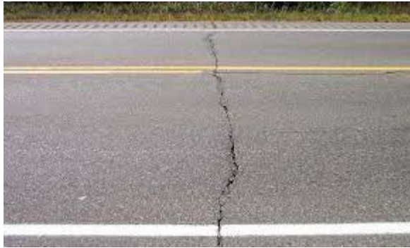
Transverse Cracking
