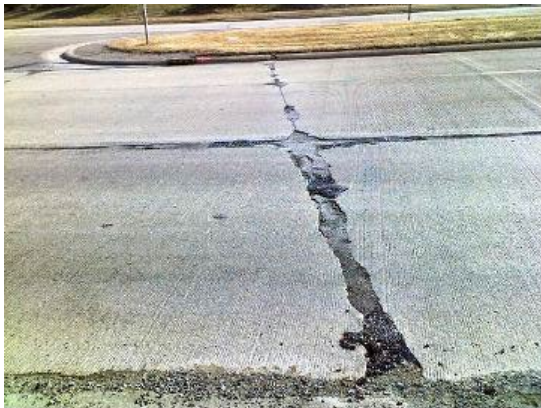
Joint Spalling/Failure
