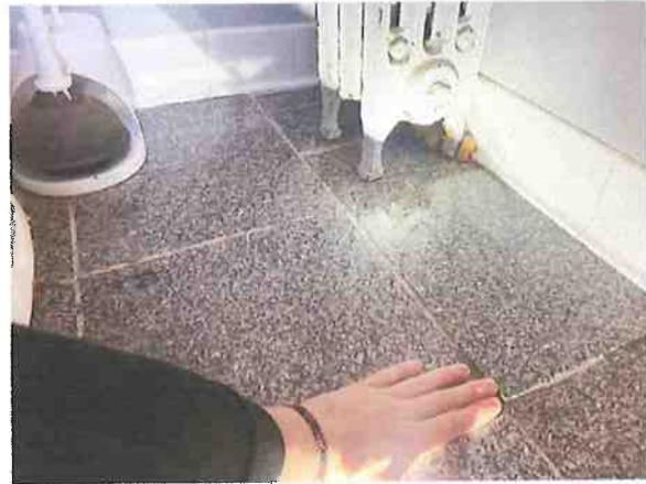
Half bathroom tiling not properly installed & unlevel
