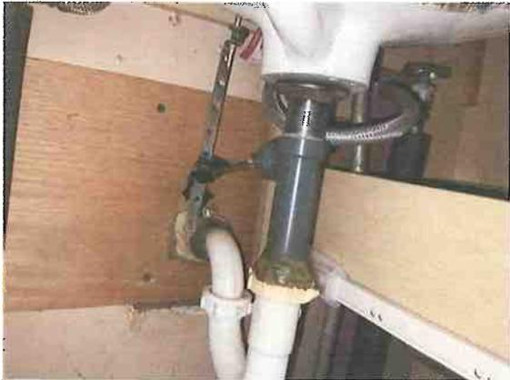
**Improper repairs master bathroom sink**
