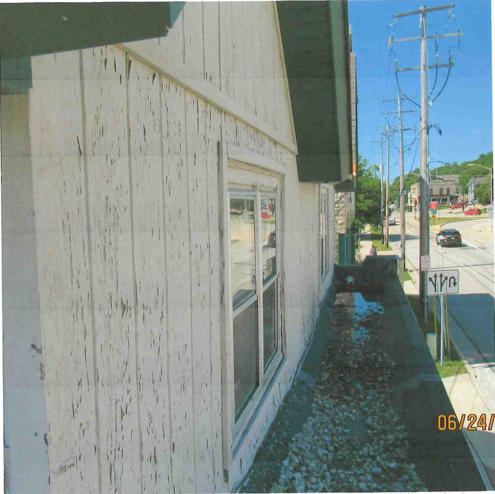
147 E. North St. Upper stone veneer – front – Phase two (2) future – next – will include new tilt-in windows
