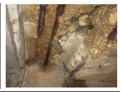
Spalled concrete in ceiling of connector to lower level.
