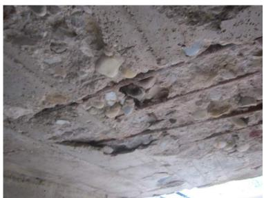
Spalled concrete in ceiling of connector to lower level.
