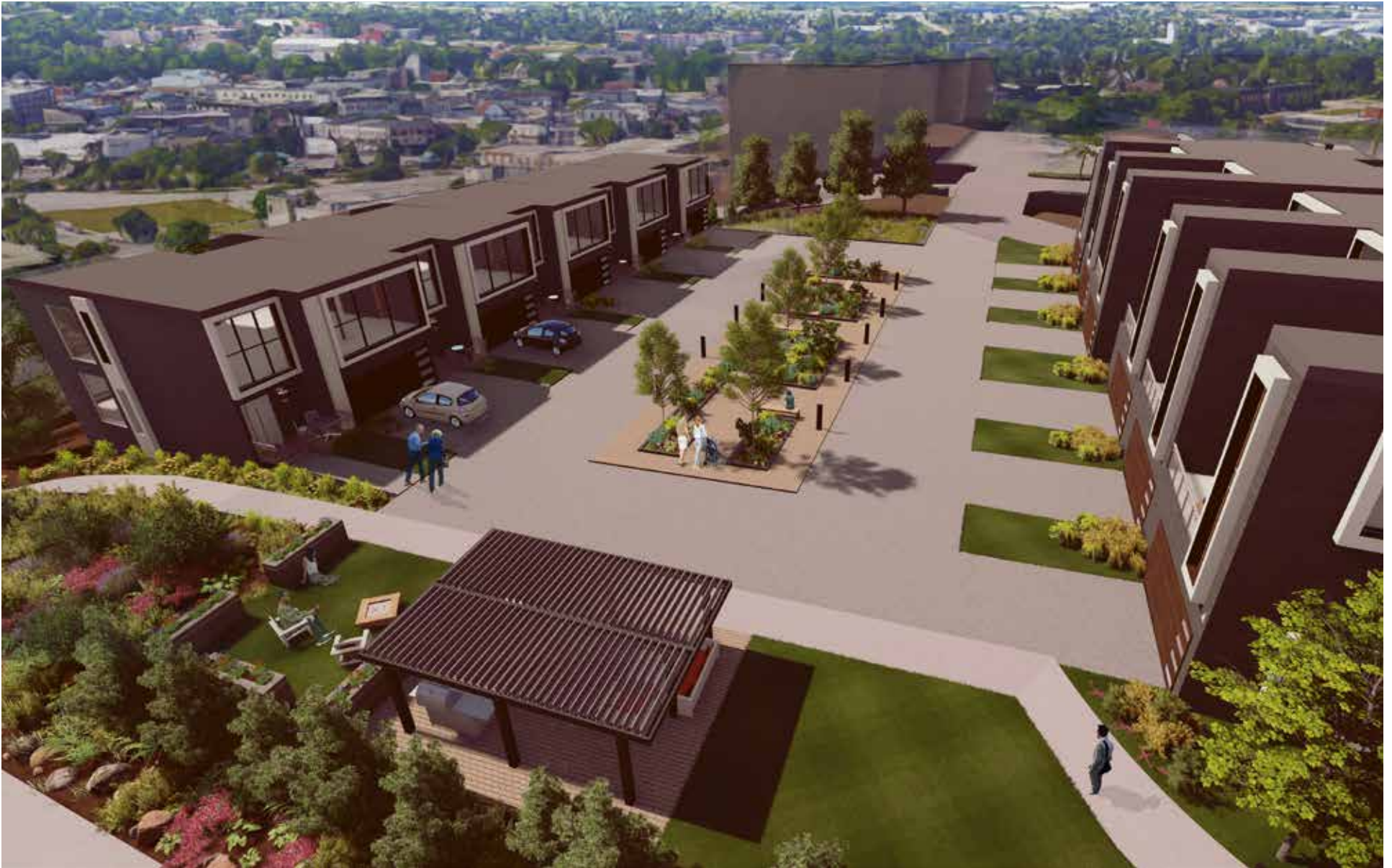
View of interior court and shared pergola, new City Hall in the background
