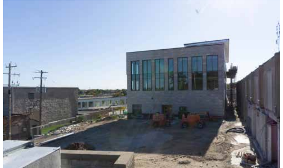
Edge condition, view of the new City Hall
