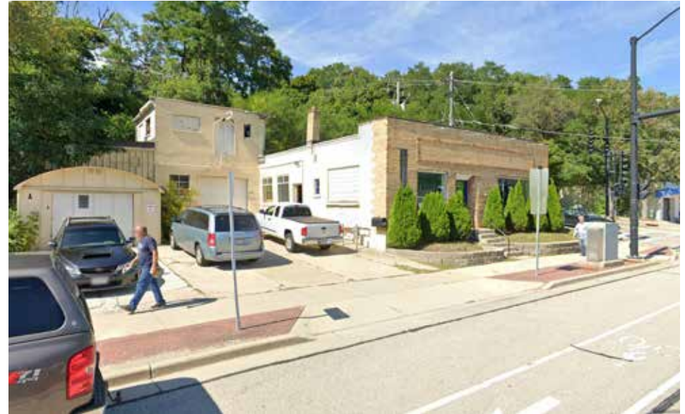
Existing buildings on North Avenue
