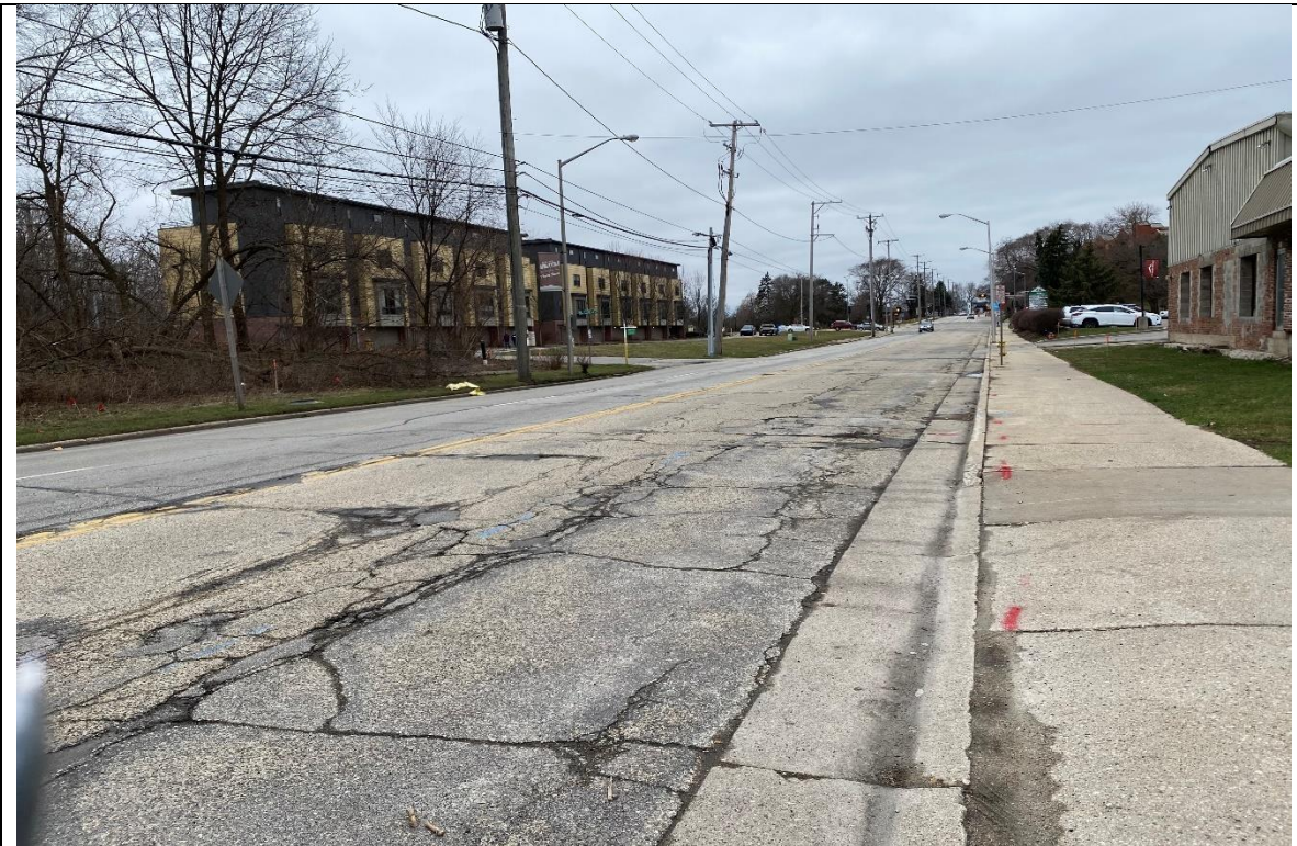
LOOKING WEST ON WEST ST. PAUL AVENUE
