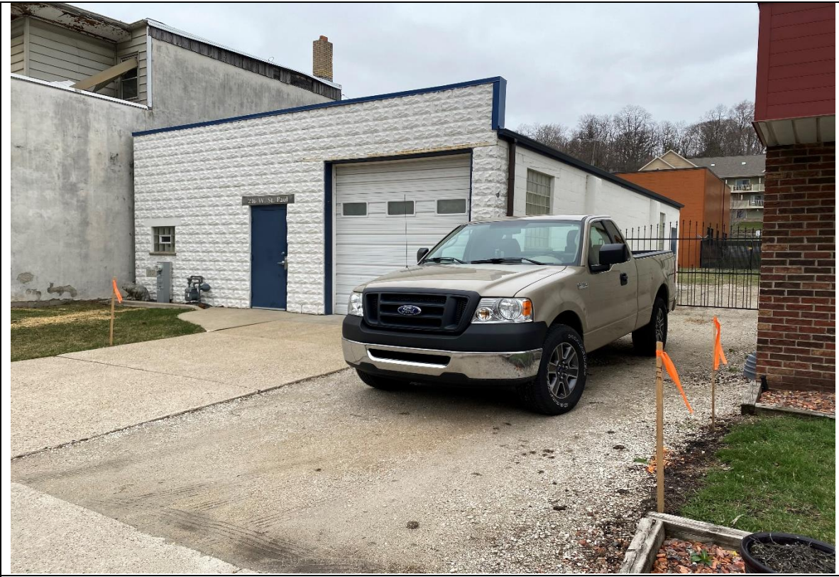
FRONT OF SUBJECT PROPERTY LOOKING NORTHWEST
