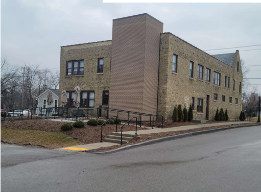
Restored West Elevation with elevator addition. View to northwest
