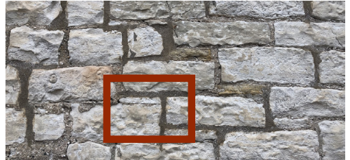
Replacement mortar should match color, texture and joint style of existing mortar.
