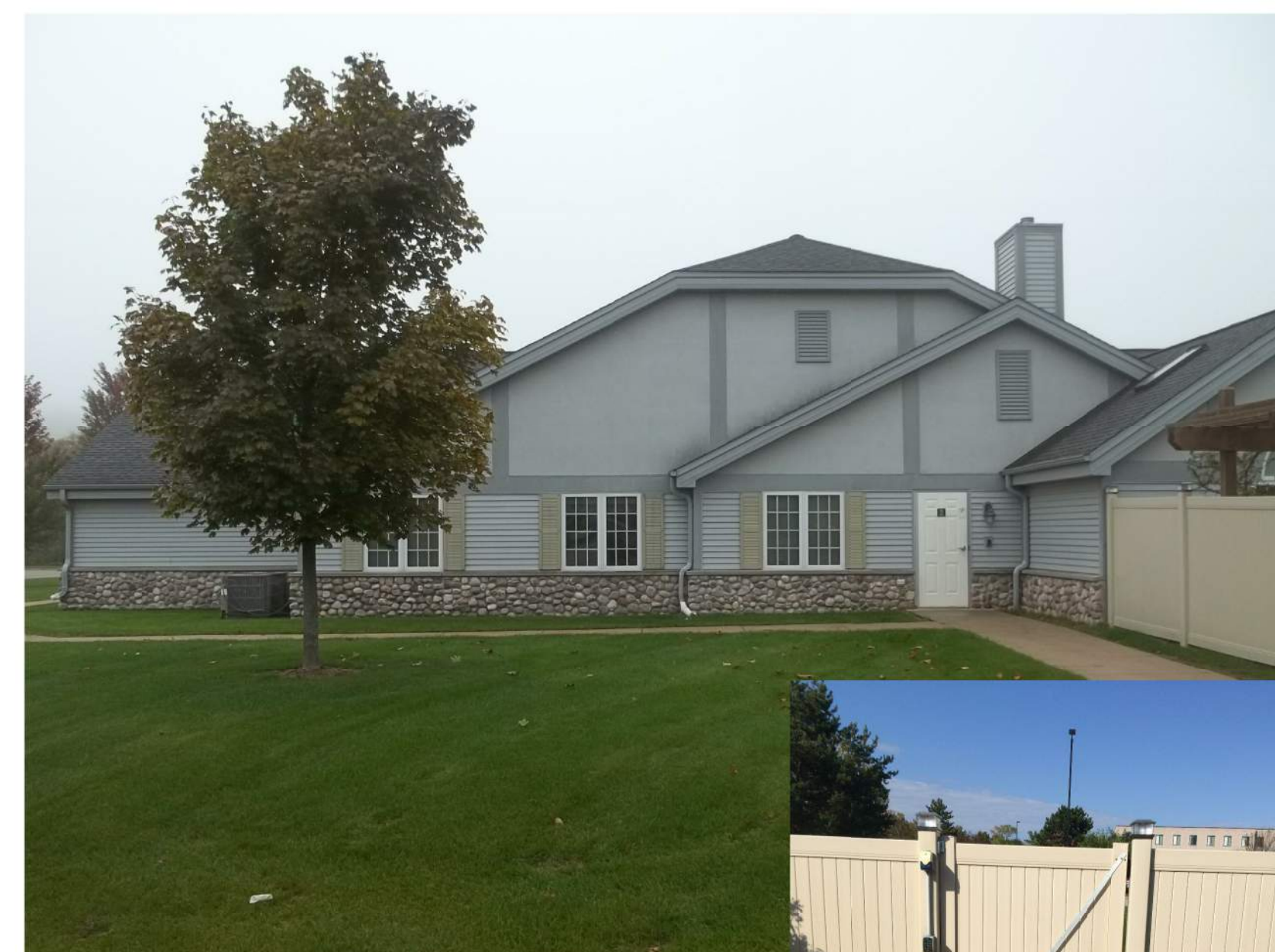
EXISTING CBRF EXTERIOR
