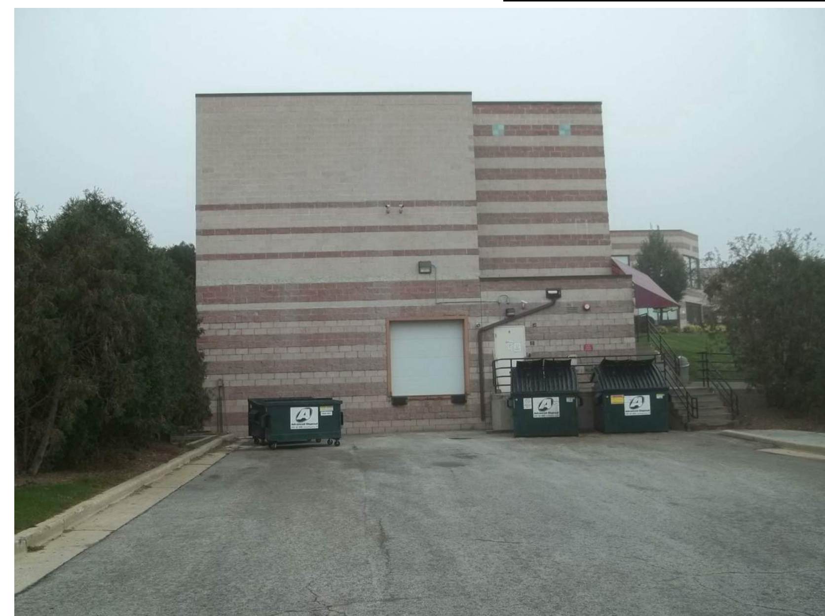
EXISTING SNF EXTERIOR (LOADING DOCK)
