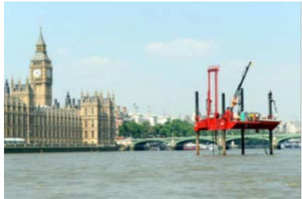
Exploration for tunnel alignment on Thames River near Palace of Westminster
