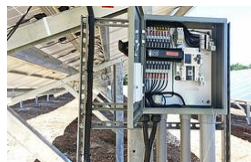
Combiner boxes and string inverters mount quickly to post using pre-punched holes
