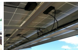
Panels mount from below or above on galvanized Z purlins which have wire management trays
