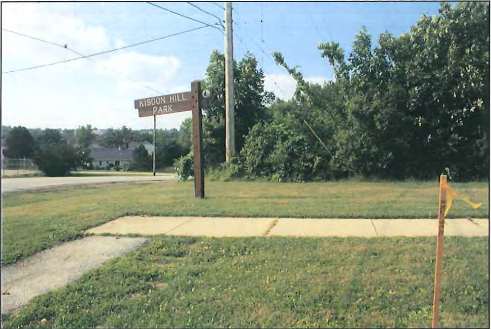
Existing Right of Way facing North and Encroaching Sign
