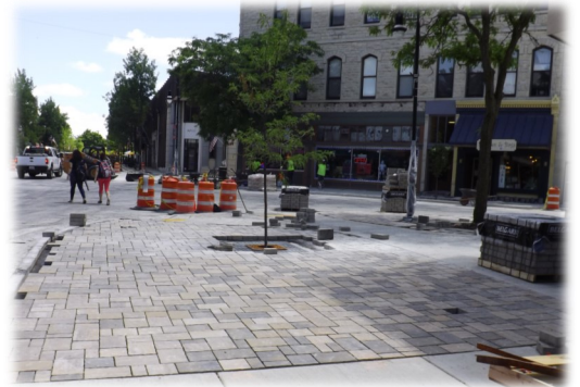
Installation of Brick Pavers
