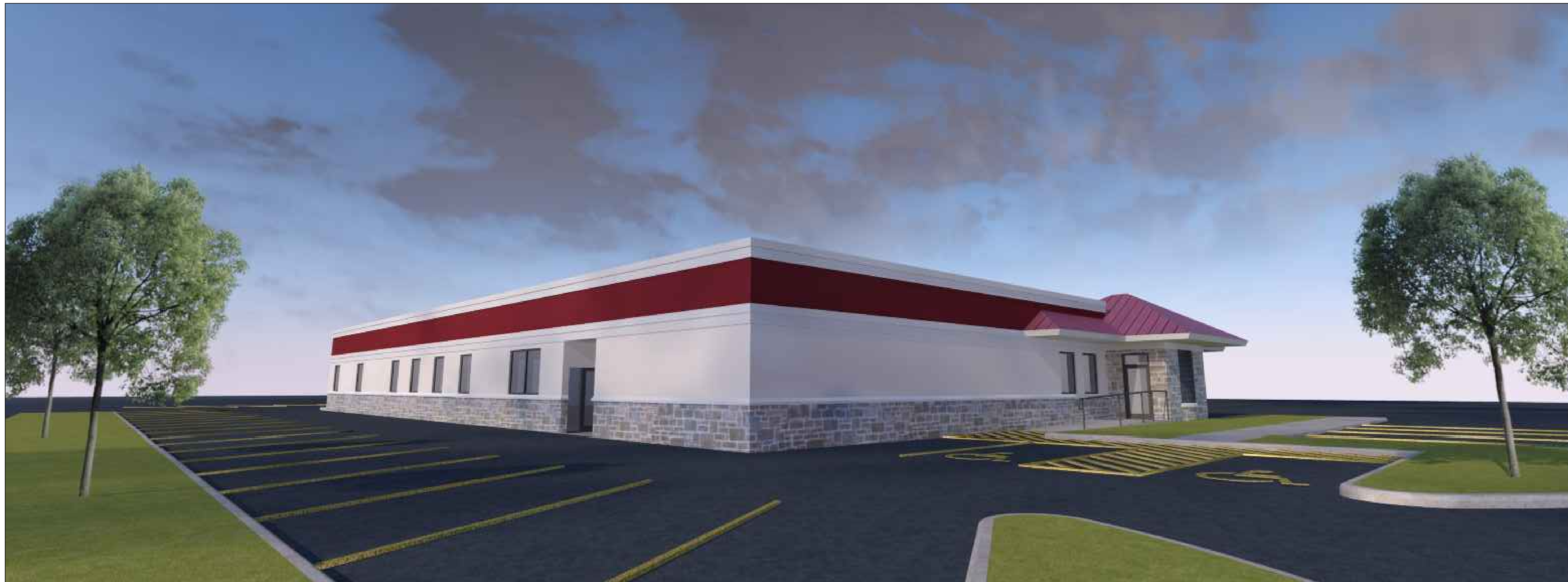
VIEW OF NORTHWEST CORNER FROM SERVICE ACCESS ROAD
