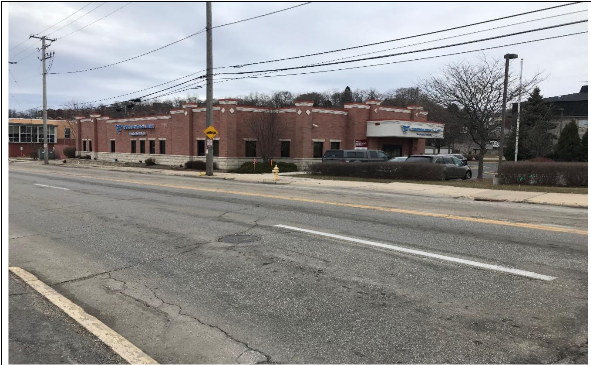
FRONT OF SUBJECT PROPERTY FROM WEST SAINT PAUL AVENUE
