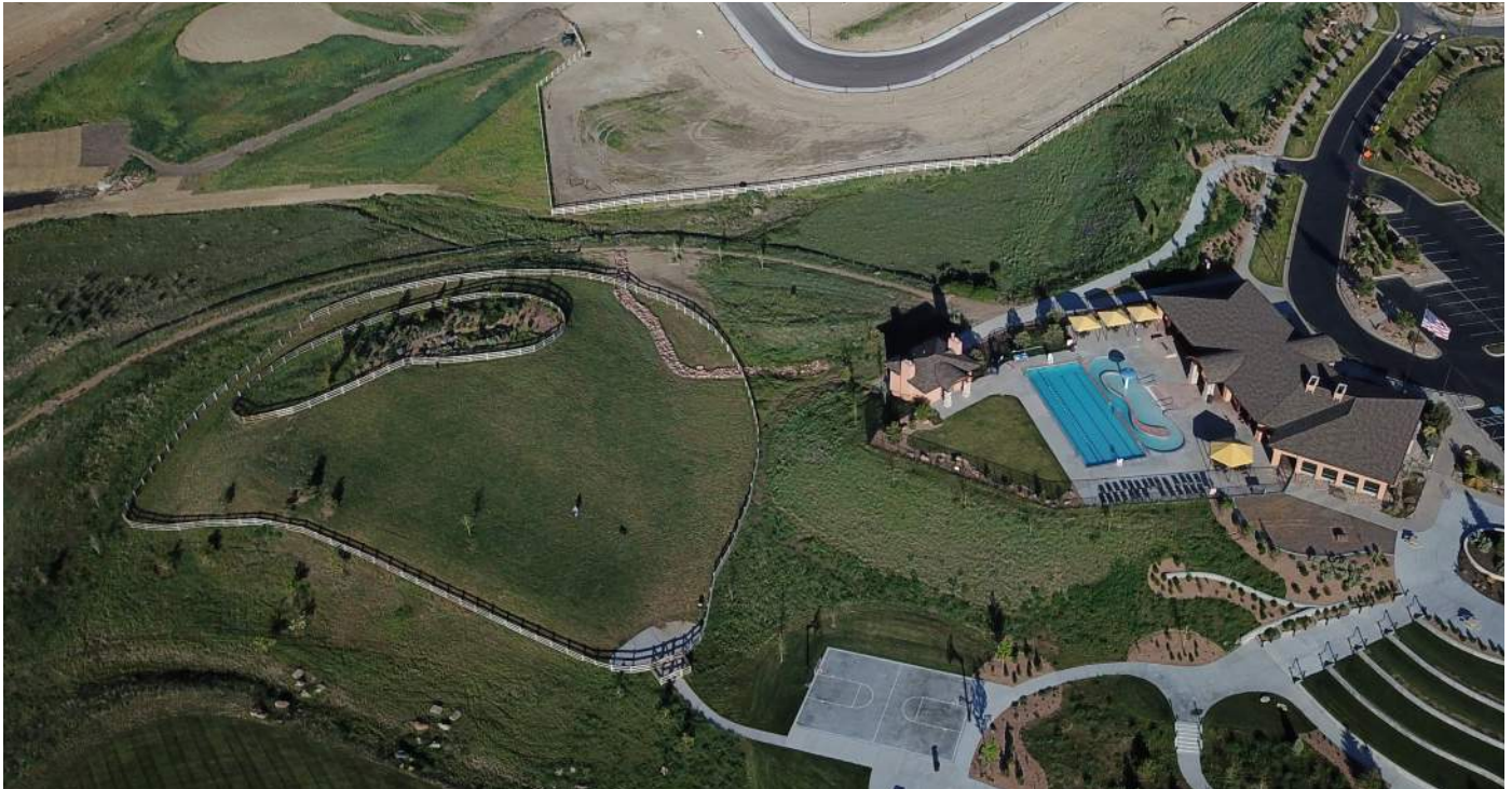
Aerial photo of Pinnacle Dog Park and recreation center.
