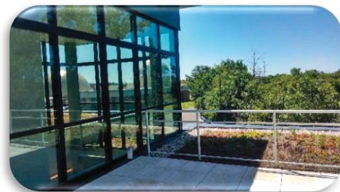
The administration building incorporated many sustainable practices including an intensive, easily accessible green roof.
