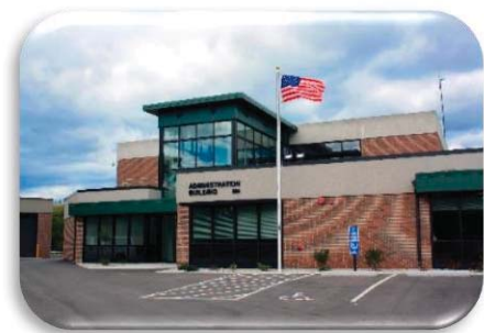
The new administration building is now a functional space for plant staff and provides a backup shelter in emergency situations for the public.
