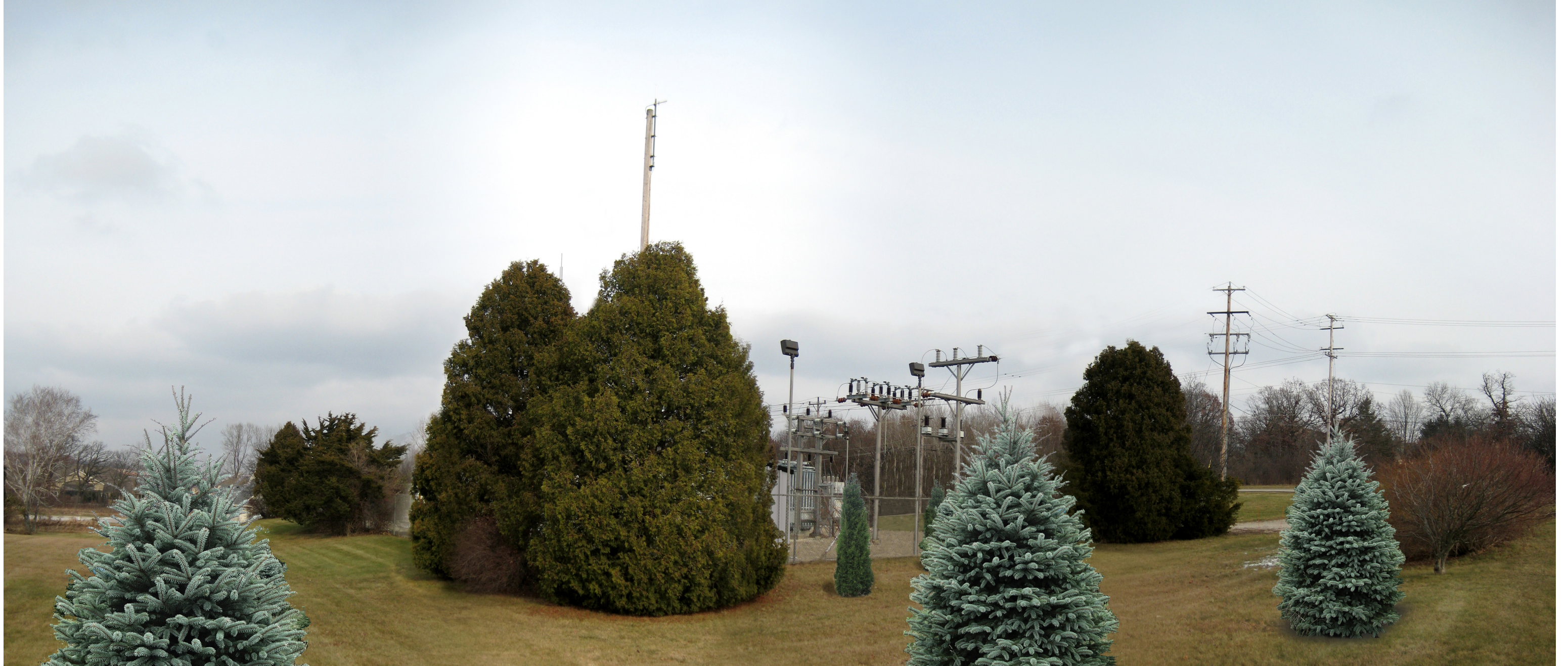
View looking Northeast after construction - 100' from substation
