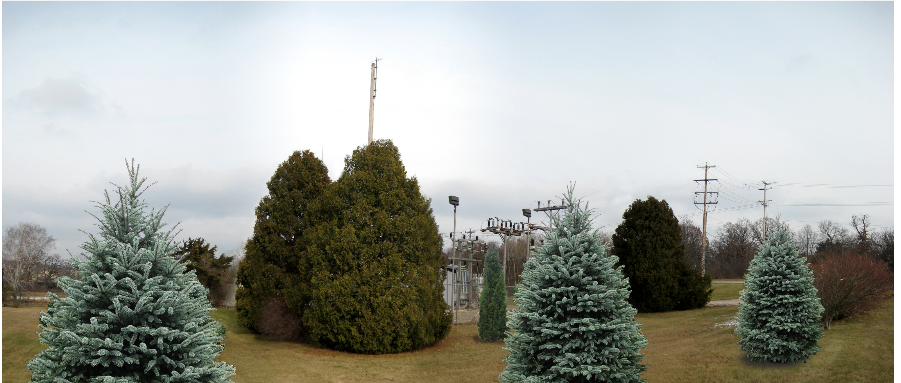
View looking Northeast after construction - 5 year growth - 100' from substation
