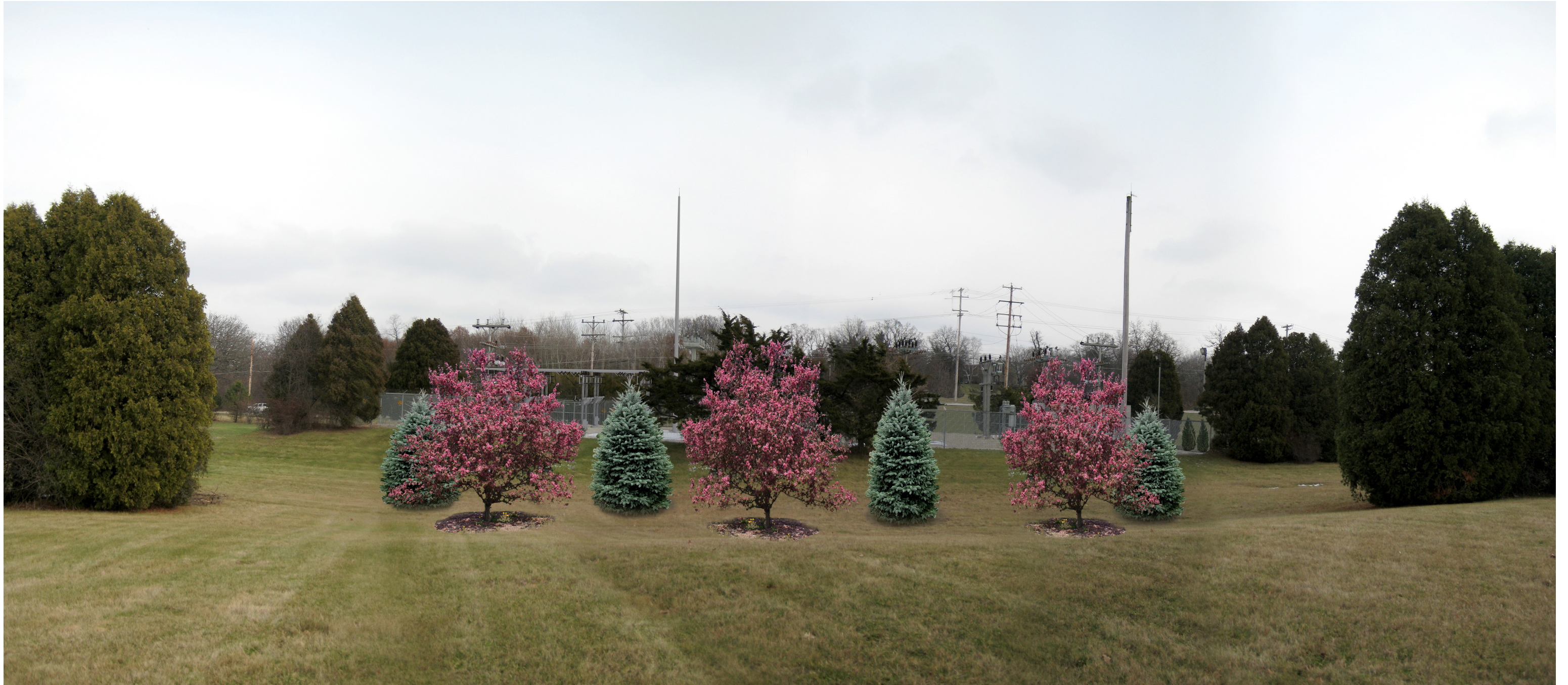
View looking East after construction - 200' from substation
