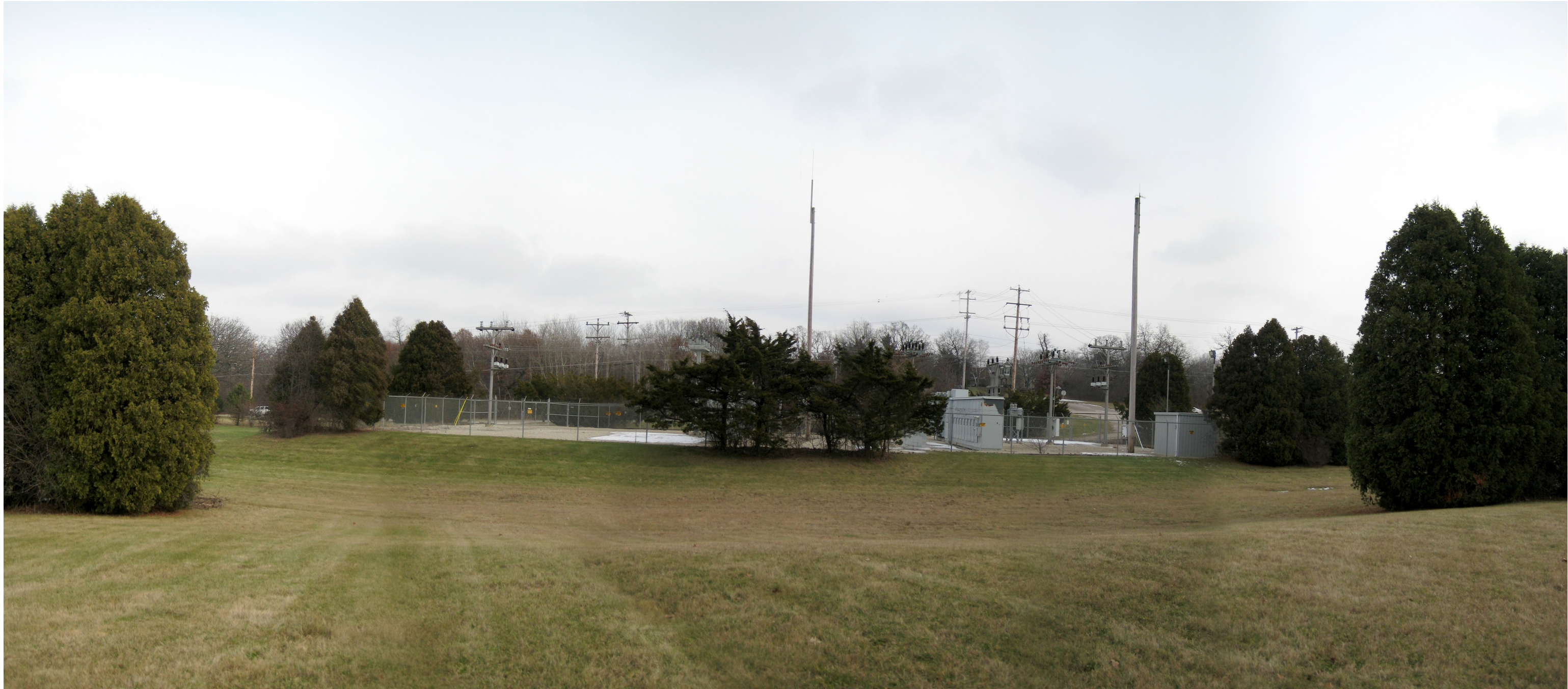
View looking East before construction - 200' from substation
