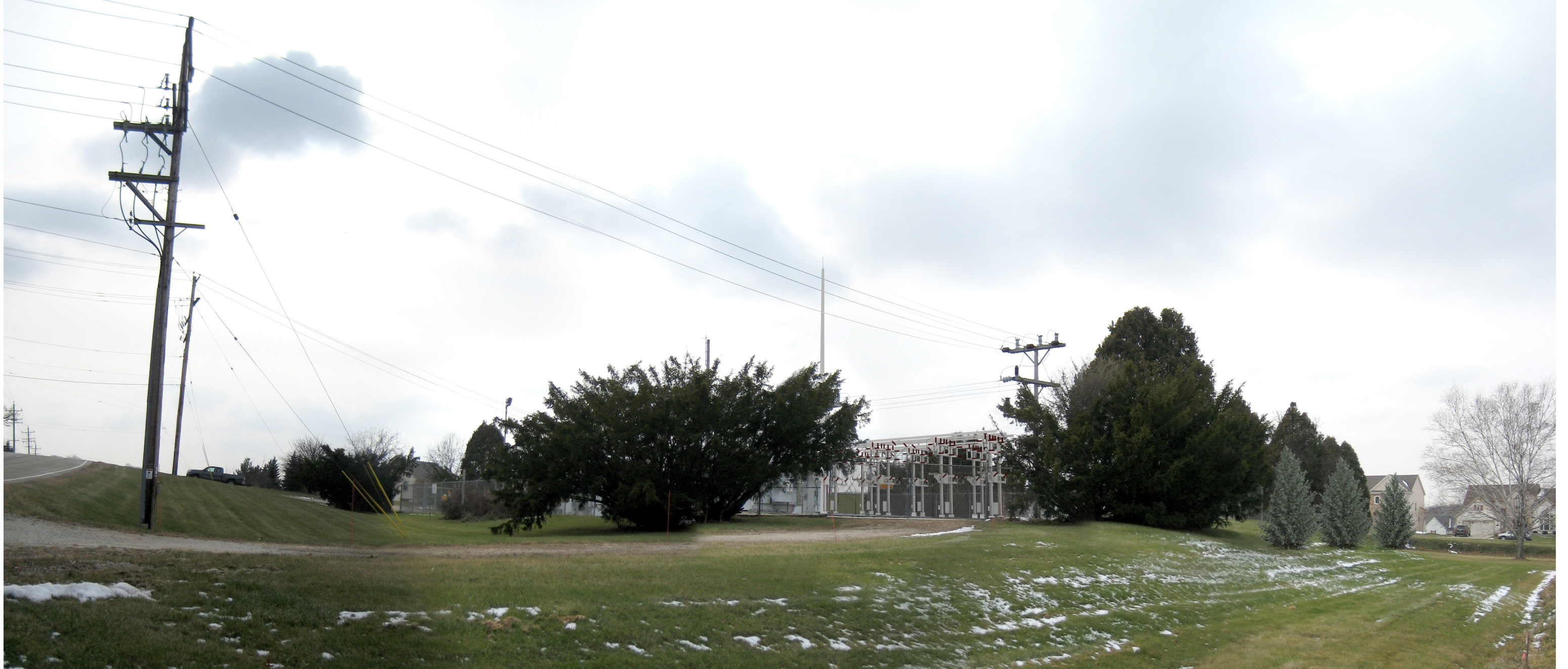
View looking Southwest after construction - 100' from substation
