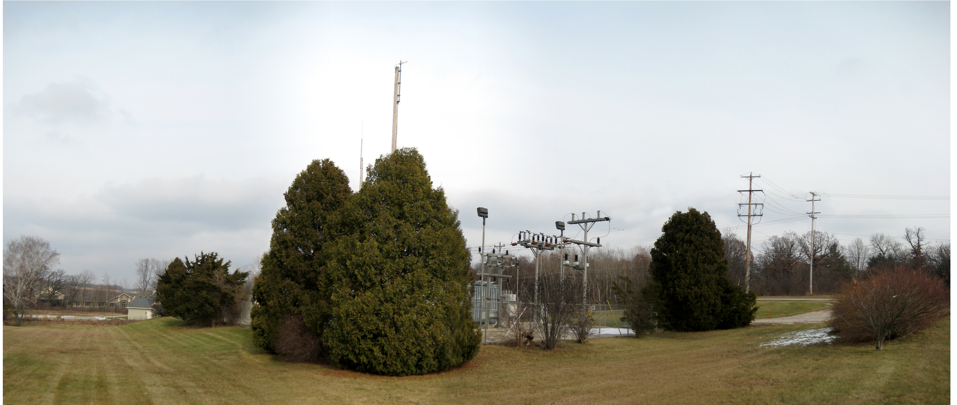
View looking Northeast before construction -00' from substation
