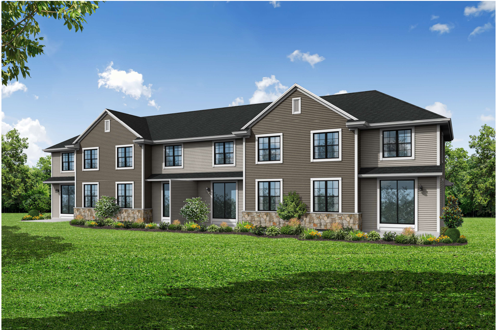
4 Unit Building – Rear Elevation – No Exposure
