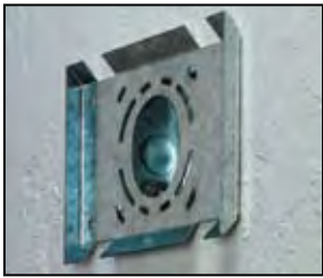
1. Attach wall-mounting plate to the junction box.
