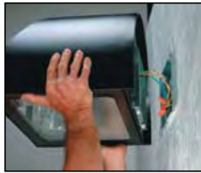
2. Make the wiring connections, and attach the fixture to the wall-mounting plate by hanging it over the beveled lip of the wall-mounting plate.
