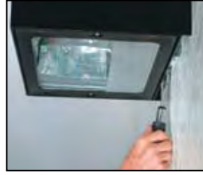
2. Make the wiring connections, and attach the fixture to the wall-mounting plate by hanging it over the beveled lip of the wall-mounting plate.
