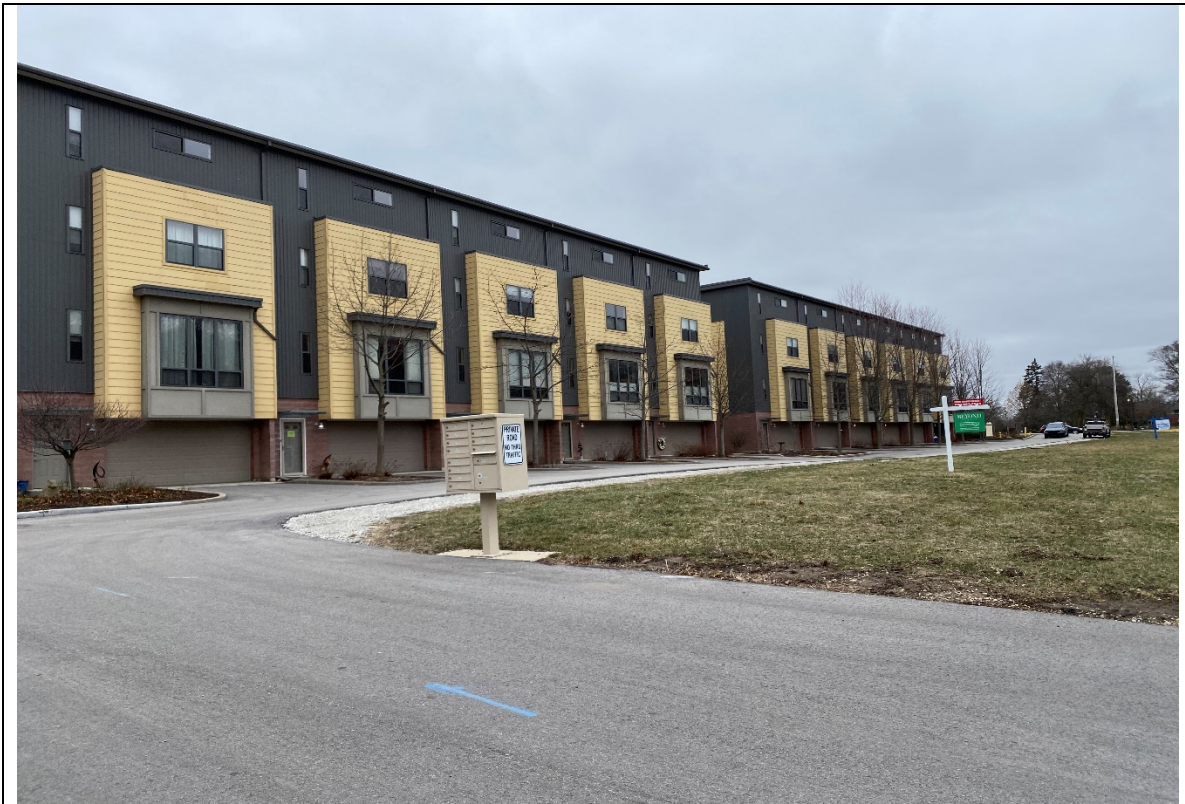
FRONT OF SUBJECT PROPERTY LOOKING SOUTHWEST
