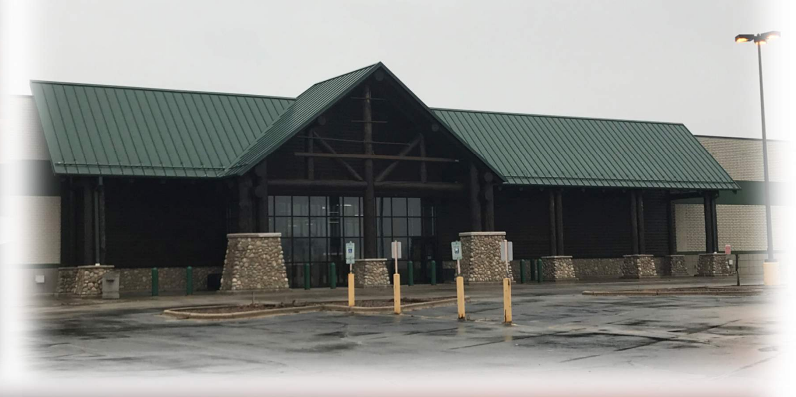
Existing Main Entry
