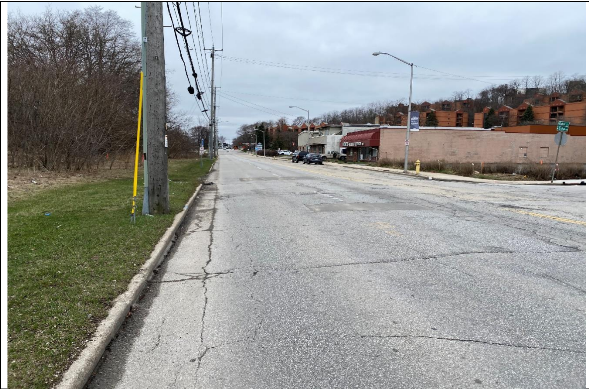
LOOKING WEST ON WEST ST. PAUL AVENUE
