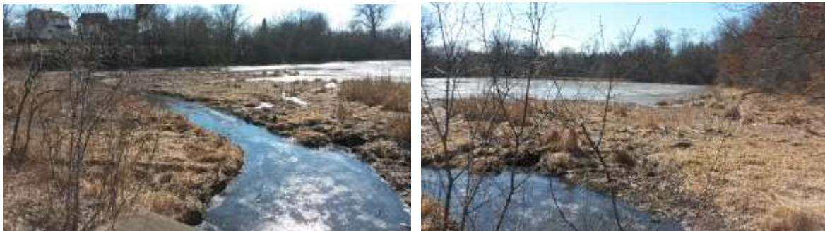
Figure 4. Sediment Plug in Woodfield Dam Pond
