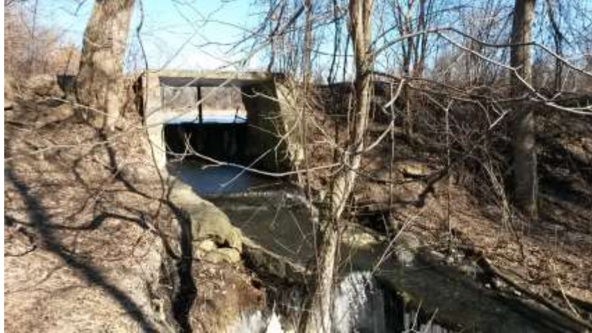
Figure 2. Woodfield Dam Outlet Structure
