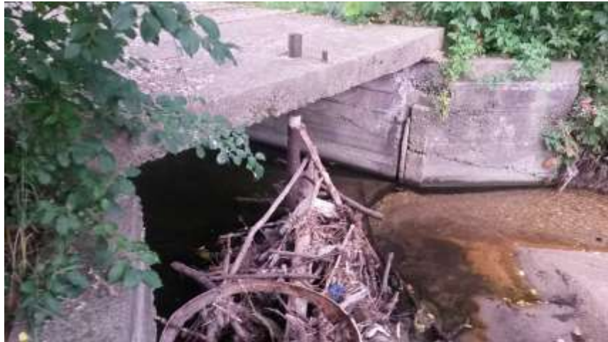
Figure 3. Woodfield Dam Pond Inlet Structure
