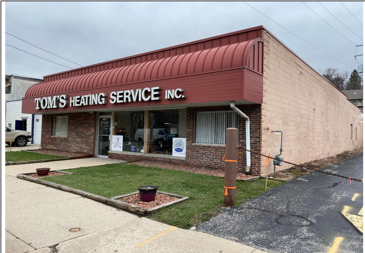
FRONT OF SUBJECT PROPERTY LOOKING NORTHWEST
