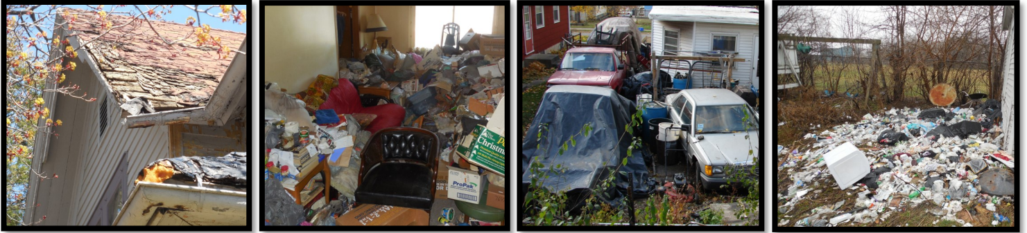
Examples of Code violations found on inspections
