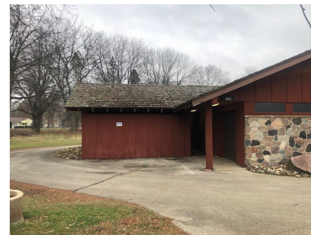
South Side Facade - Before
