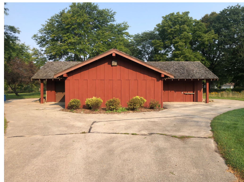
Parking Lot Facade - Before
