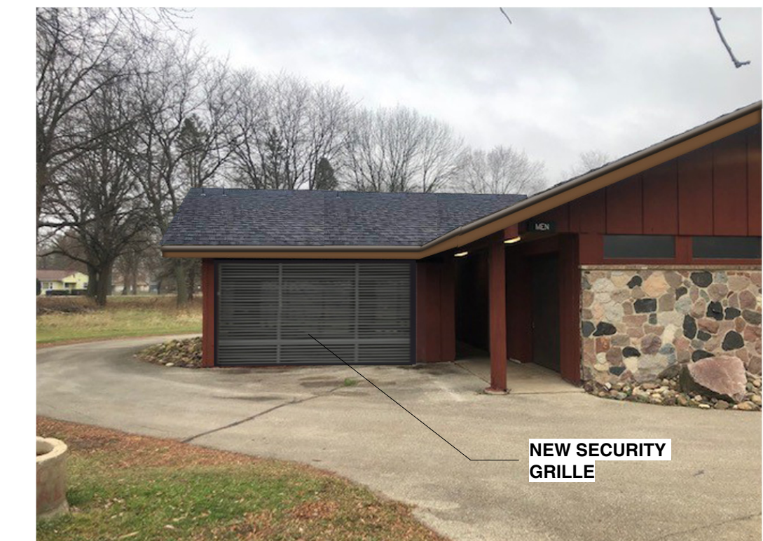
South Side Facade - After
