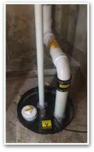
Once the sump crock is sealed, we can start our piping directly from the sump crock, or we can core a hole in the floor and tap into the drain tile (helpful for system placement).
