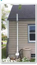
home. The piping must continue all the way up the outside of the home and vent above the roofline at least 12" to comply with EPA standards. We keep the system aesthetically pleasing by running it near pre-existing vertical lines when possible. We also strive to position the system towards the back or back corners of the home, and/or behind landscaping when possible.
