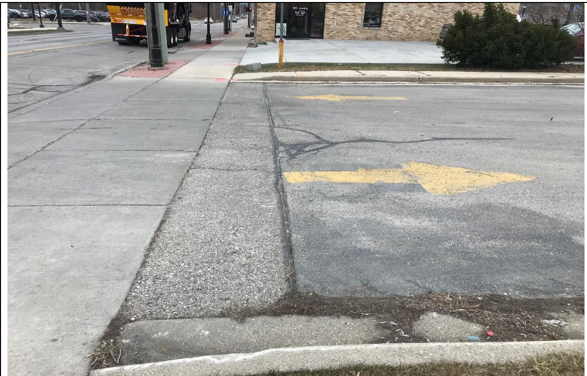
TLE LOOKING SOUTHWEST ALONG EAST SAINT PAUL AVENUE
