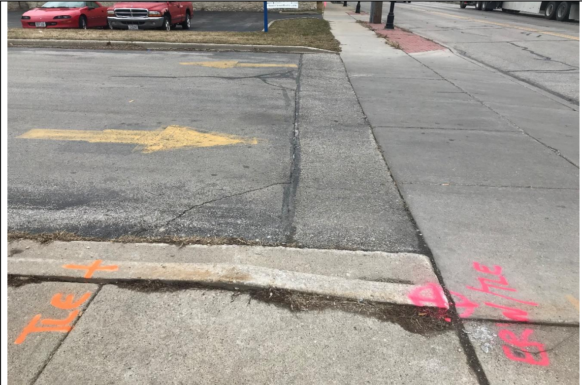
TLE LOOKING NORTHEAST ALONG EAST SAINT PAUL AVENUE
