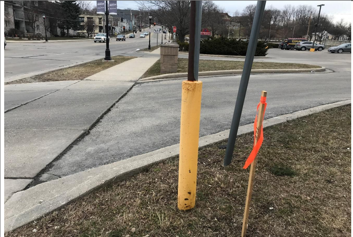
TLE AND PLE LOOKING NORTHWEST ALONG MADISON STREET
