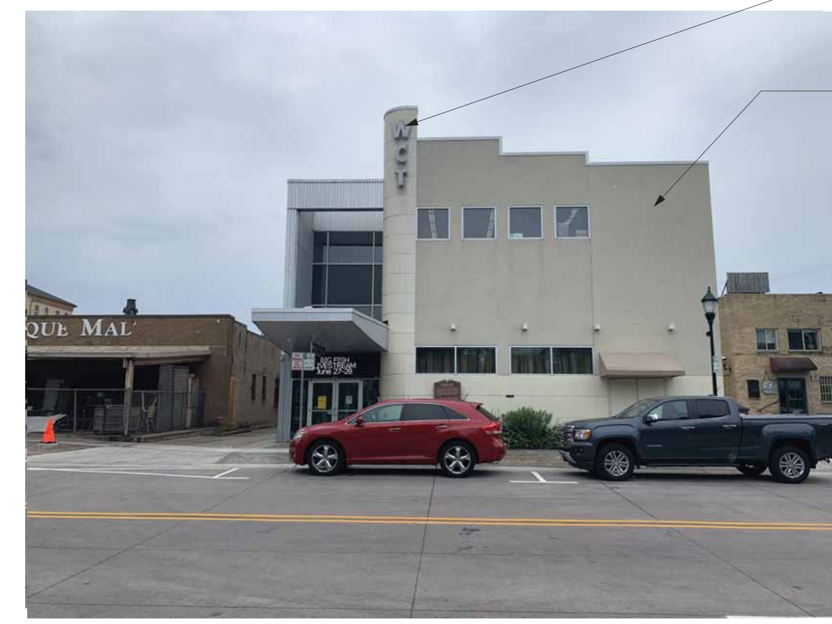
EXISTING BACK EXTERIOR OF THEATRE - ASSUME MINOR MAINTENANCE
