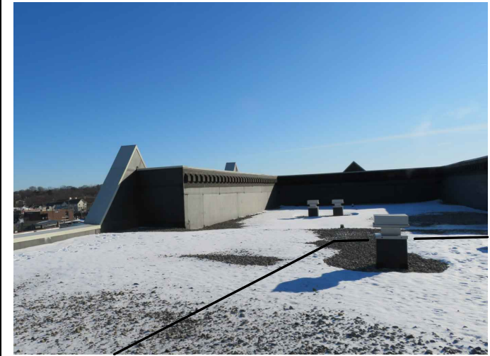
3 PROPOSED COAX ROUTE ACROSS ROOF SCALE: N.T.S.
