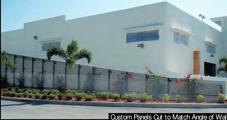
Custom Panels Cut to Match Angle of Wall
