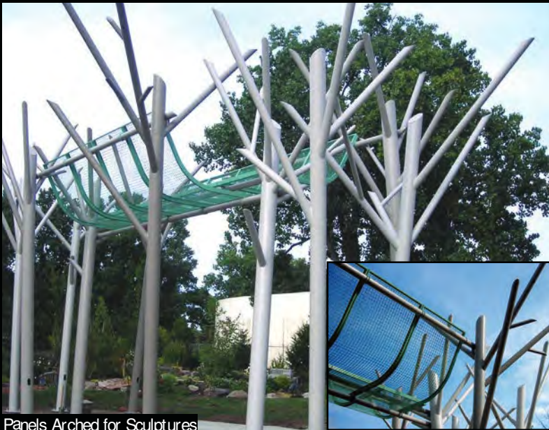
Panels Arched for Sculptures
