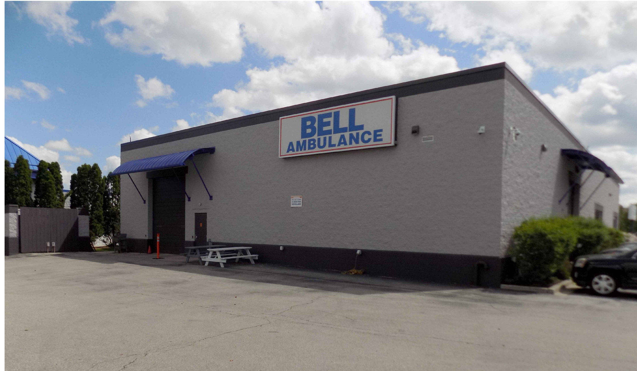
3 COLOR PHOTO OF EXISTING EXTERIOR FINISHES SCALE: NO SCALE
