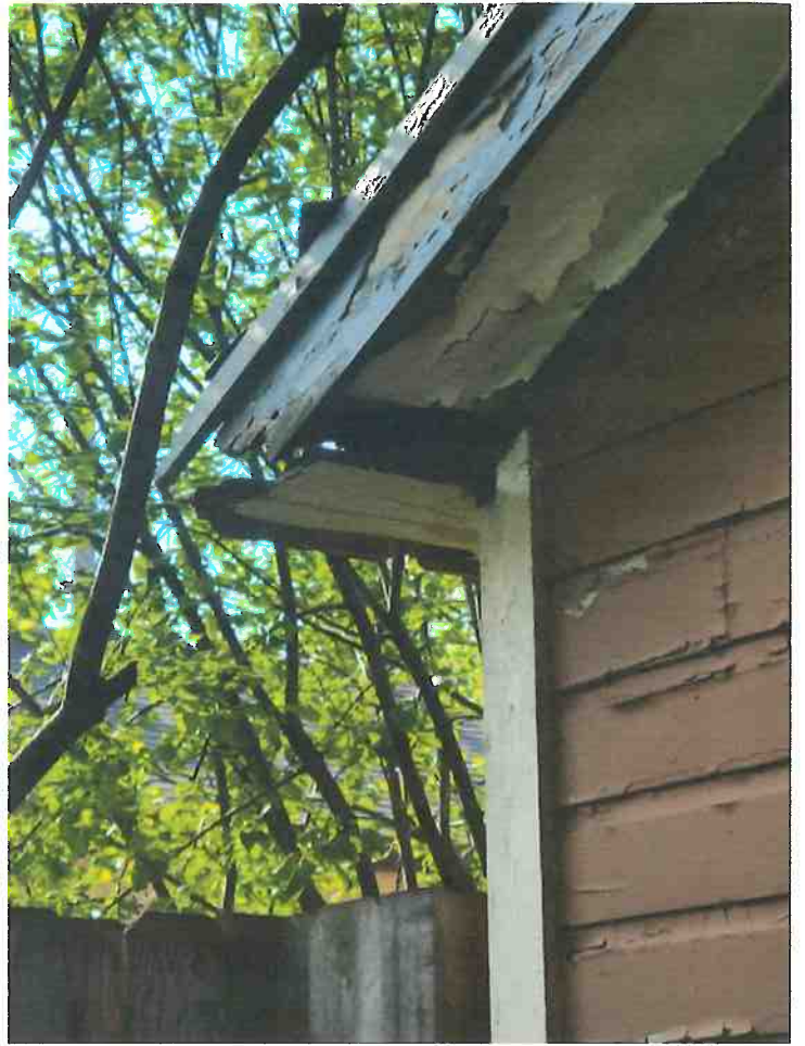
Rotted Fascia & Soffit
