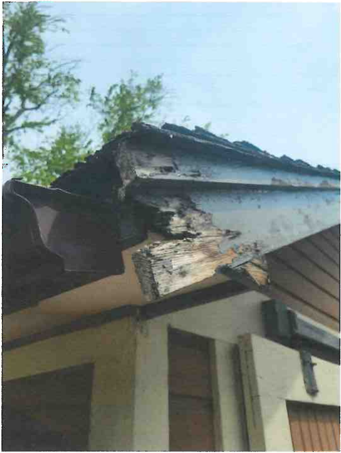
Rotted Fascia & Soffit
