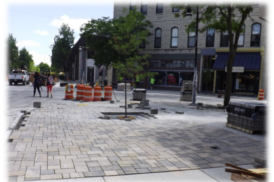
Installation of Brick Pavers
