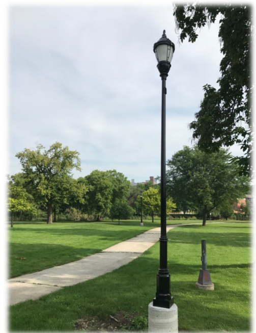
New LED lights installed at Bethesda Park
