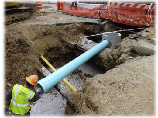
Installation of Storm Sewer
