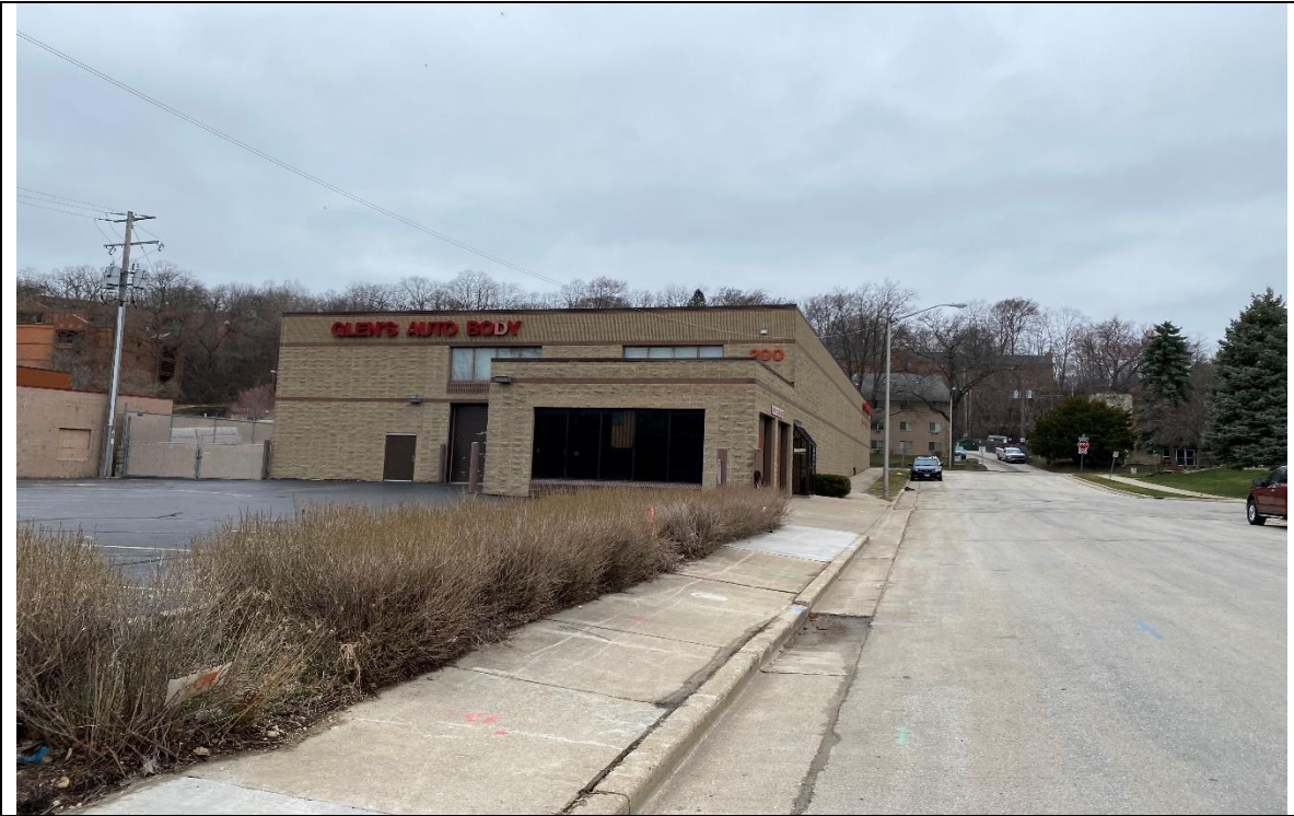
FRONT OF SUBJECT PROPERTY LOOKING NORTH
