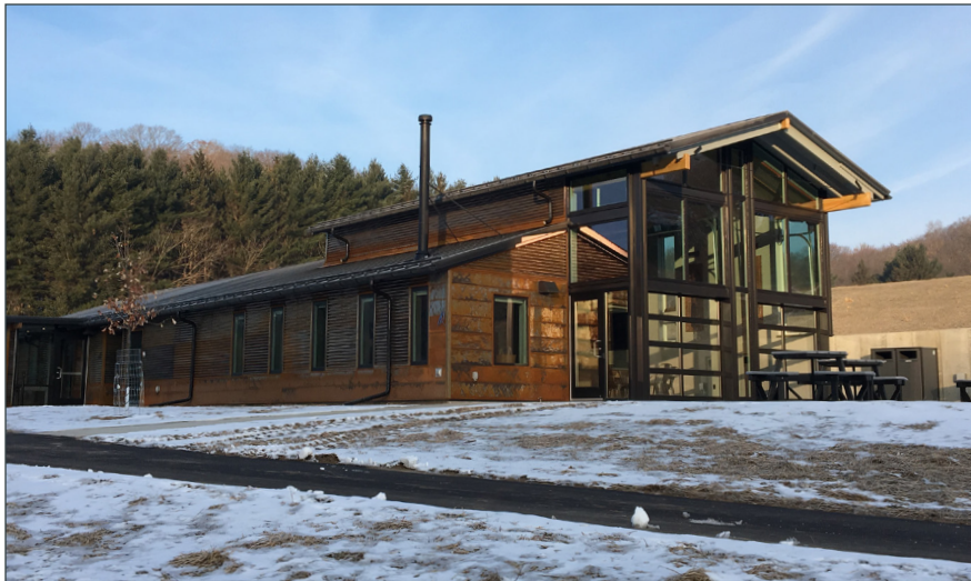
Clad in Corten steel, the building will weather to a deep brown color.
